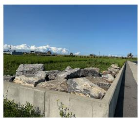
Photo 9: Cover system repair made at top of retaining wall at the southern portion of the Site, looking north. The displaced surge stone was moved back in to place and covered with large rip-rap stone.
