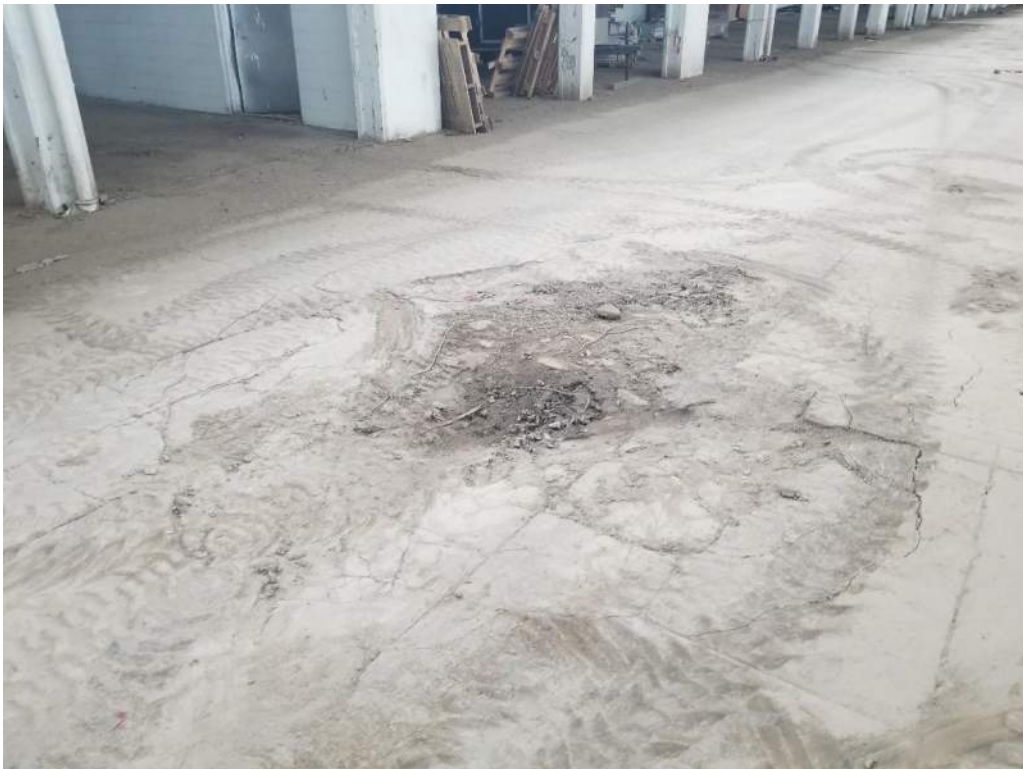
View of damaged concrete floor inside Garage Building.
