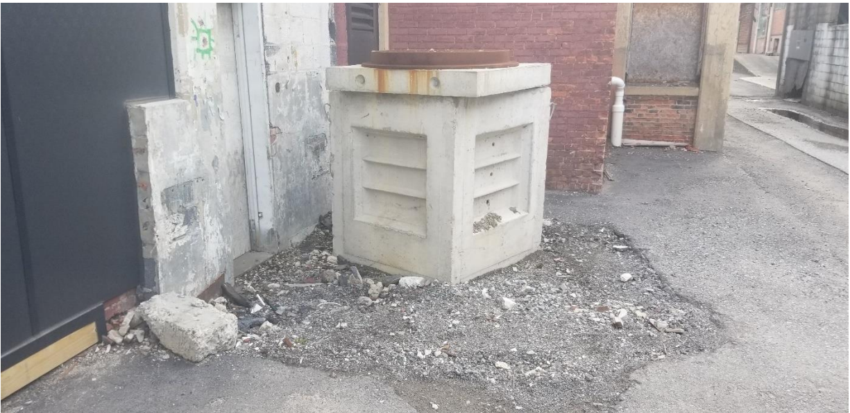
View of new storm water catch basin staged to be installed.
