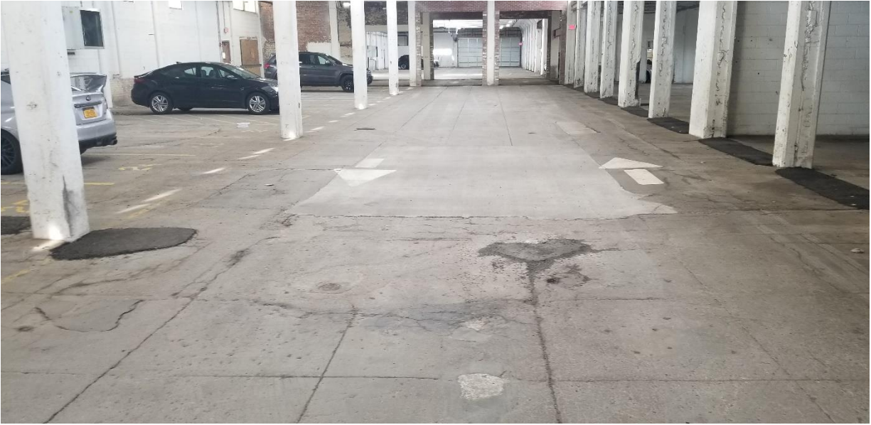
View of repaired concrete floor inside Garage Building.
