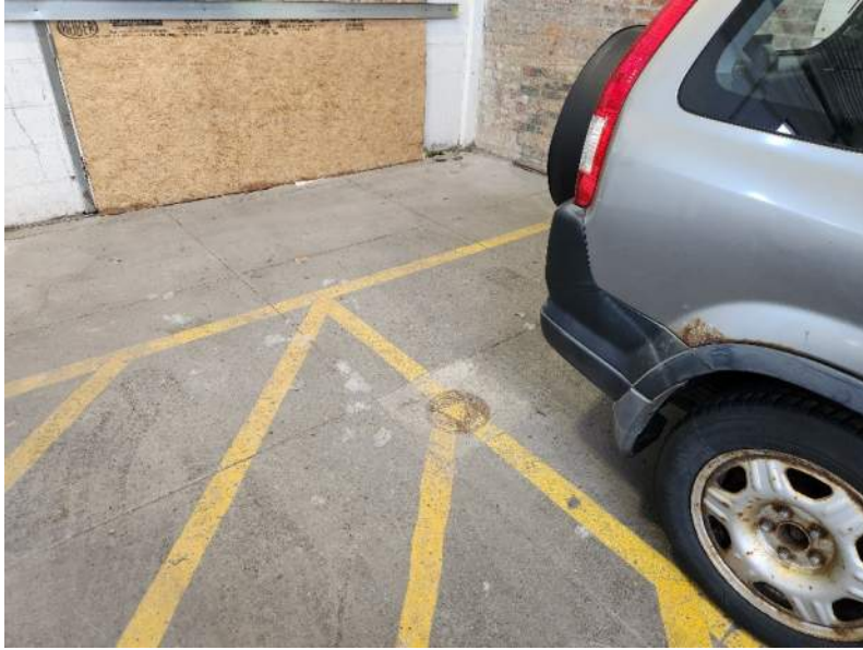
View of monitoring well inside the Garage Building.
