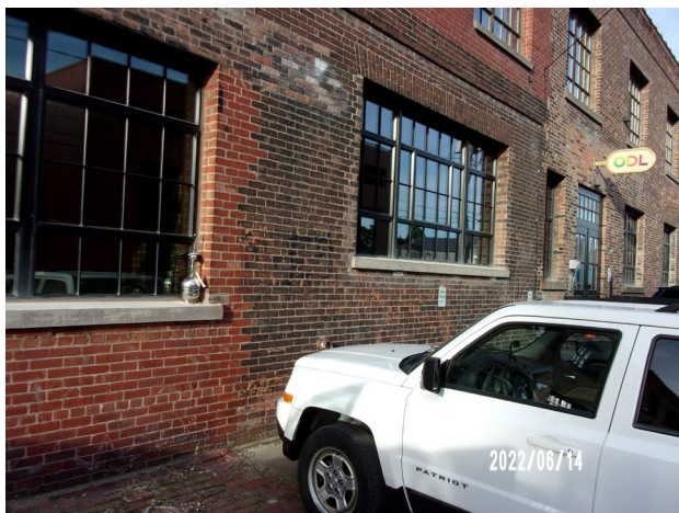
1. View of OA-2(061422) near the northern exterior of the structure.
