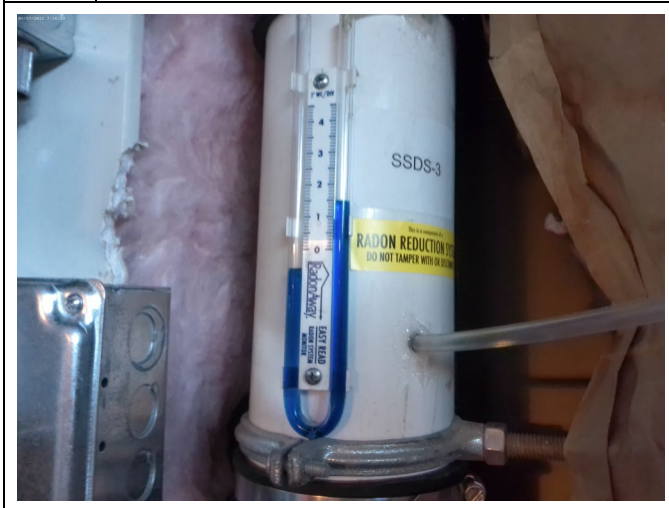
5. 12/19/22 – View of SSDS #3 Manometer Enclosure
