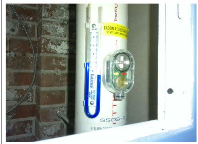
3. 12/19/22 – View of SSDS #2 Manometer Enclosure
