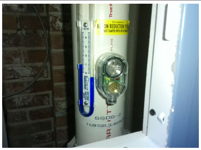
4. 12/19/22 - View of SSDS #2 Manometer Reading
