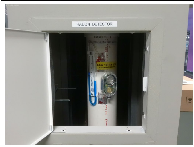
1. 12/19/22 – View of SSDS #1 Manometer Enclosure
