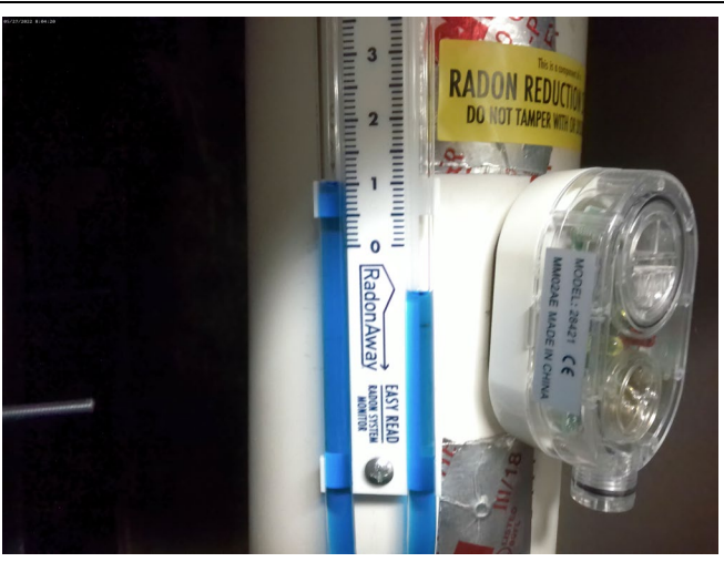
2. 12/19/22 - View of SSDS #1 Manometer Reading
