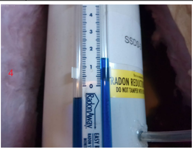
6. 12/19/22 - View of SSDS #3 Manometer Reading
