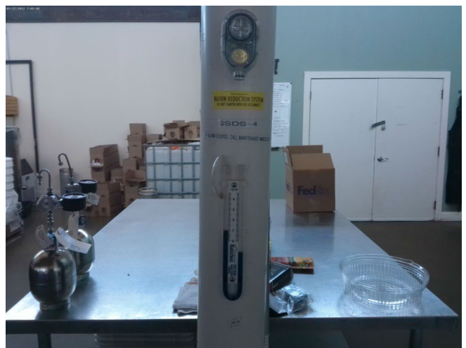
8. 12/19/22 – View of SSDS #4 (not enclosed)
