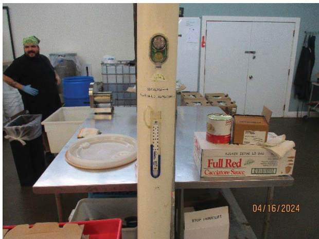
9. View of SSDS #4 (not enclosed).
