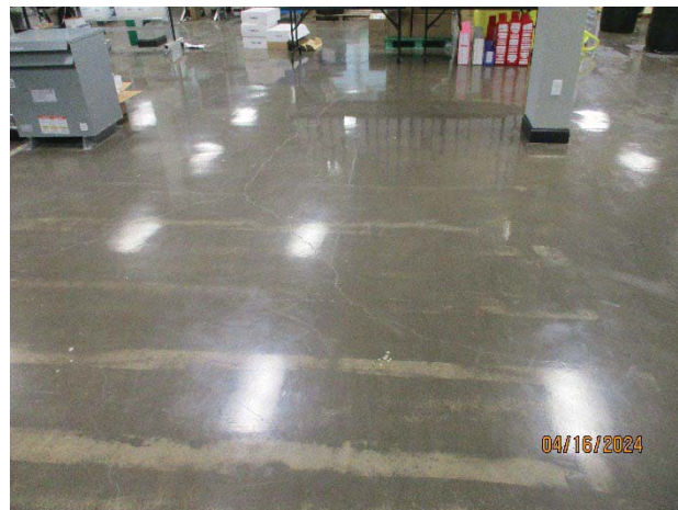
10. View of the cover around SSDS #1 facing east.
