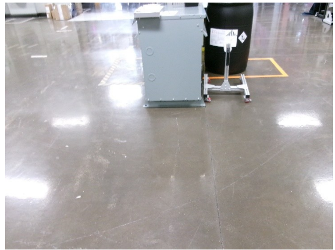
18. 1/13/25 – View of floor in the vicinity of SSDS-1.
