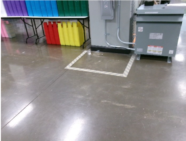
19. 1/13/25 – View of floor in the vicinity of SSDS-1
