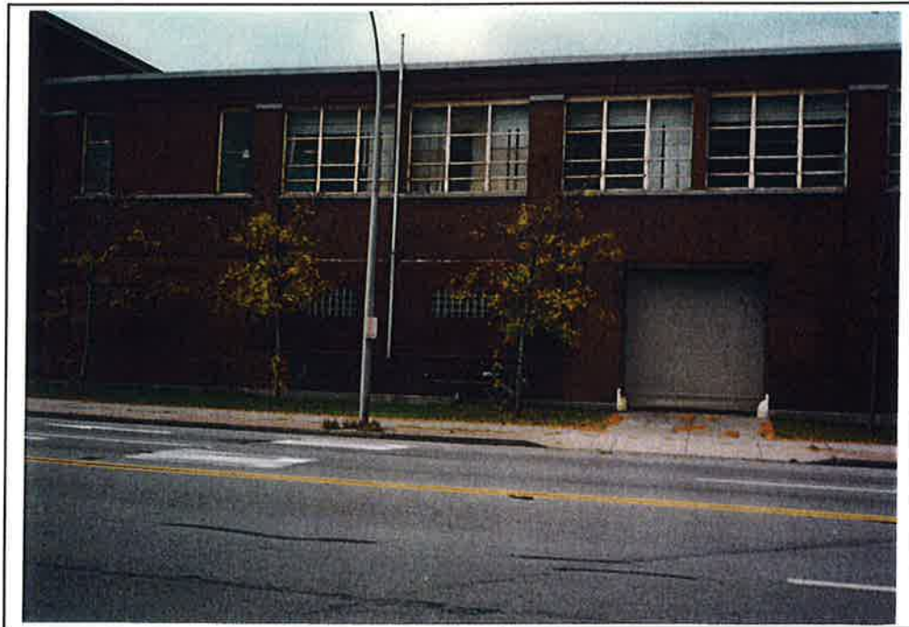
East side of building along Niagara Street
