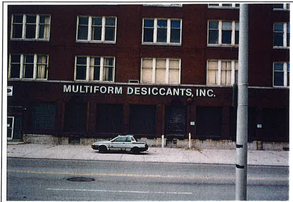
East side of building along Busti Avenue
