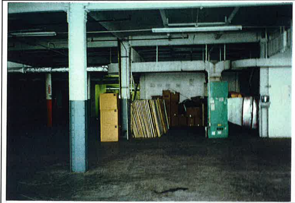
Fourth floor, open area west of offices, view east 960 Busti Avenue
