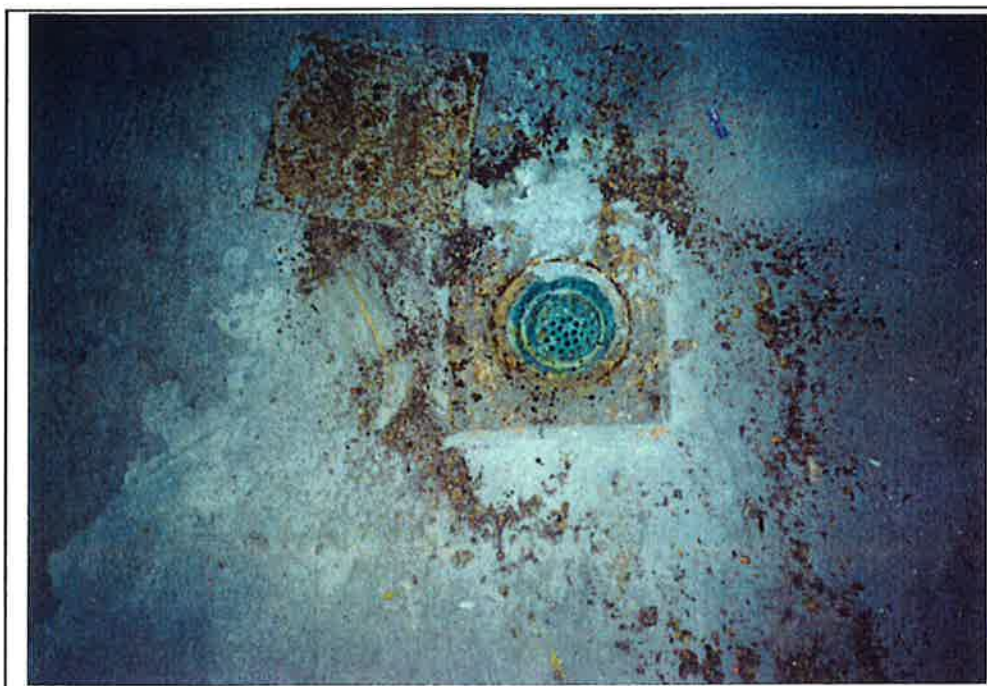
Basement, floor drain
