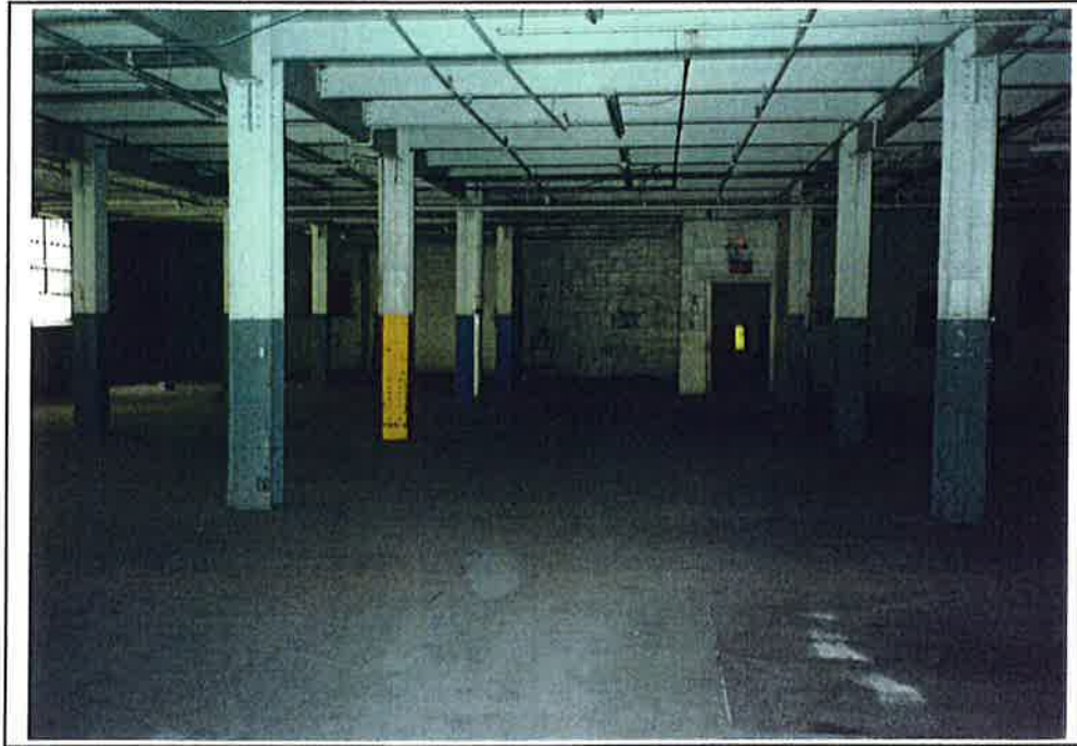
First floor, view north
