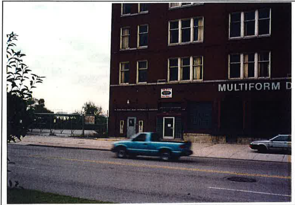
East side of building along Busti Avenue
