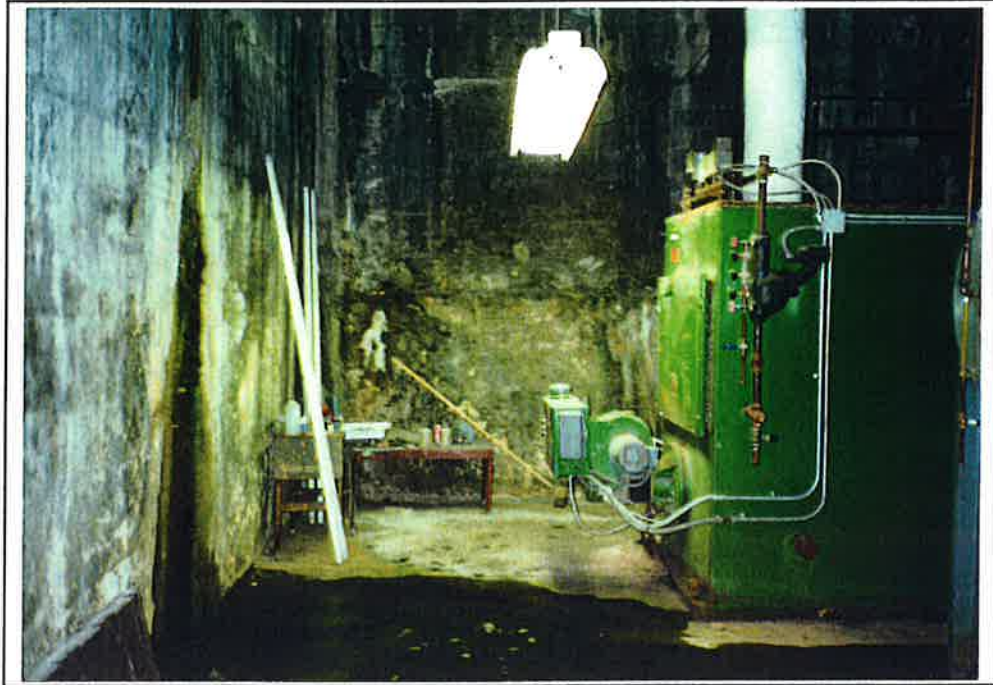
Sub-basement, view east along north wall
