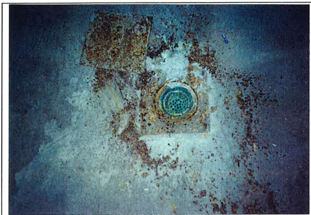
Basement, floor drain
