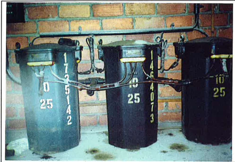
Basement, 10 kVA transformers
