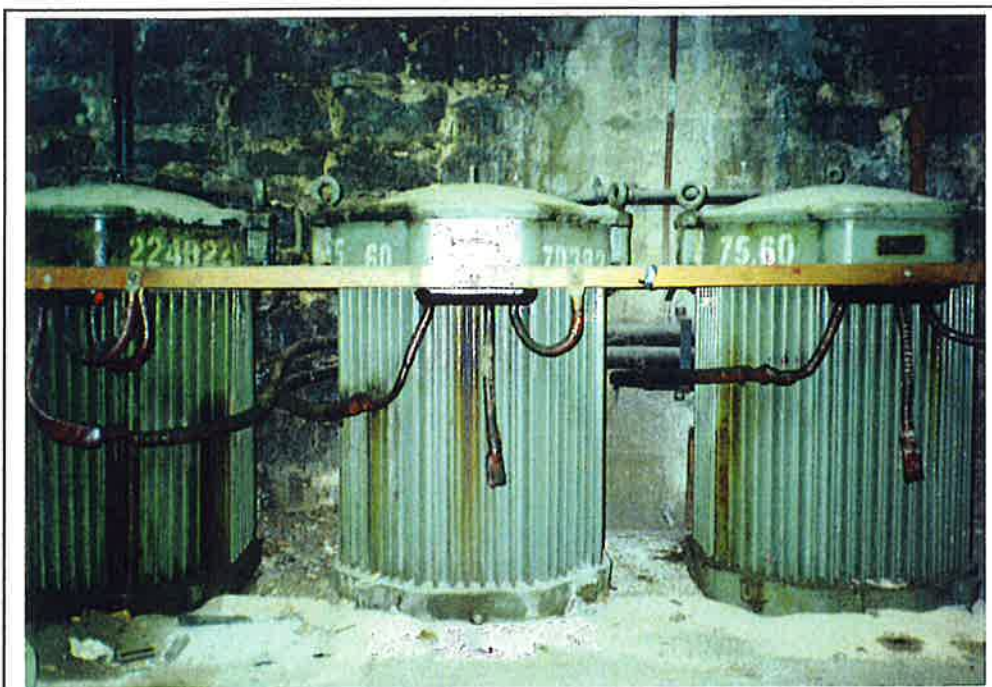
Basement, 75 kVA transformers
