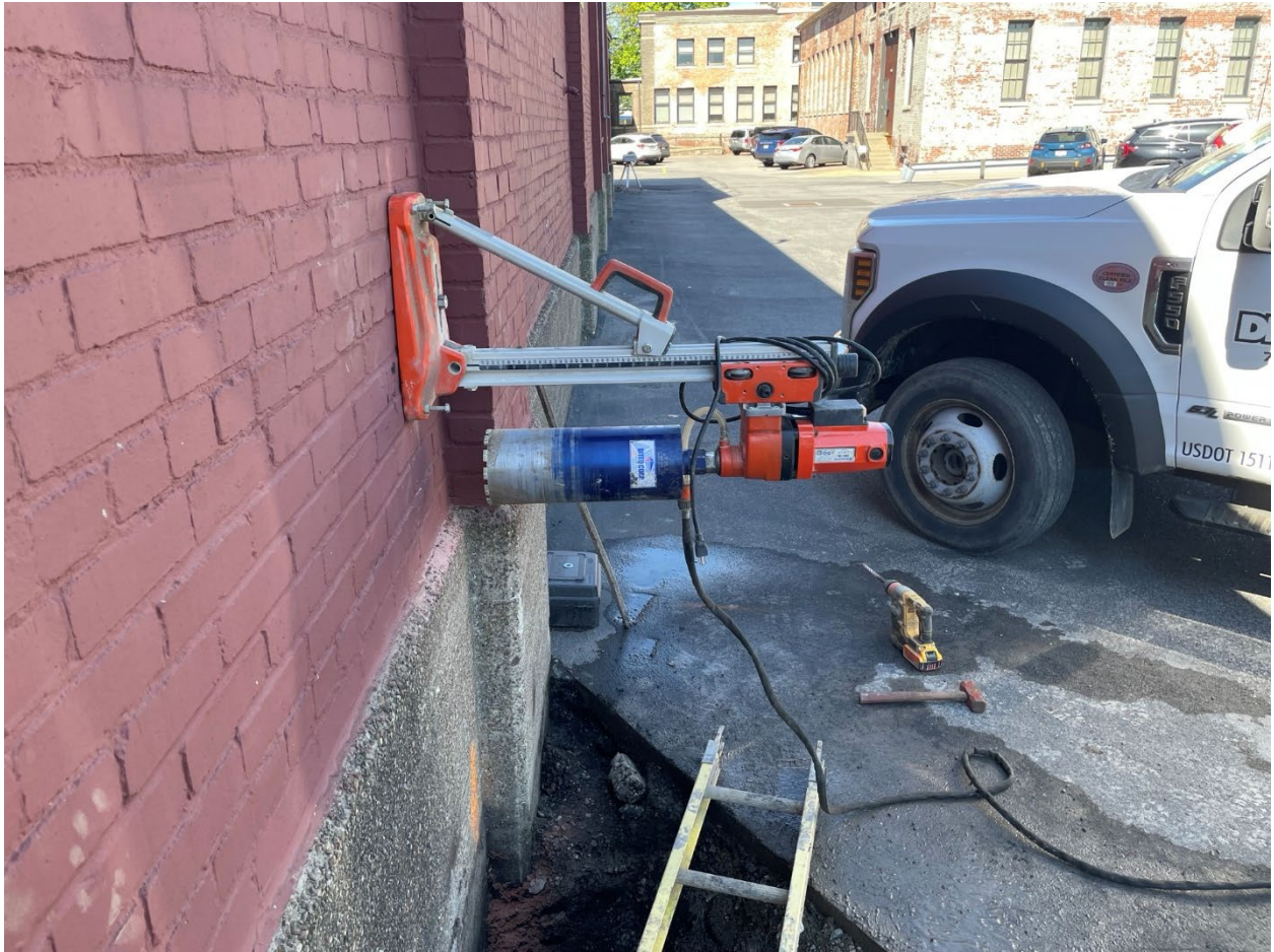
Area where 4-inch roof drain connection will exit the building.
