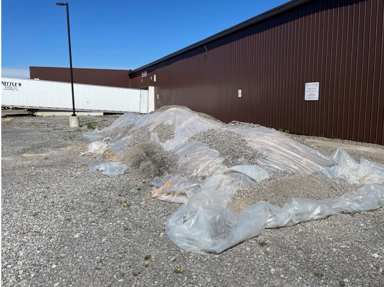
Spoils stockpile at southern site area.
