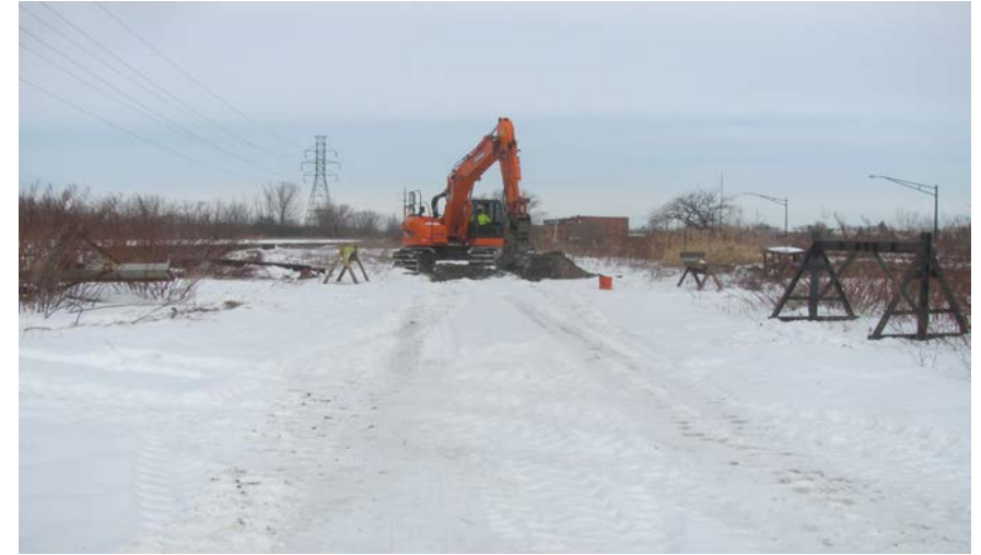
54. View of location of Test Pit- TP-1 facing north
