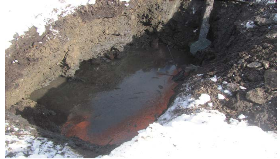
62. View of completed TP-3
