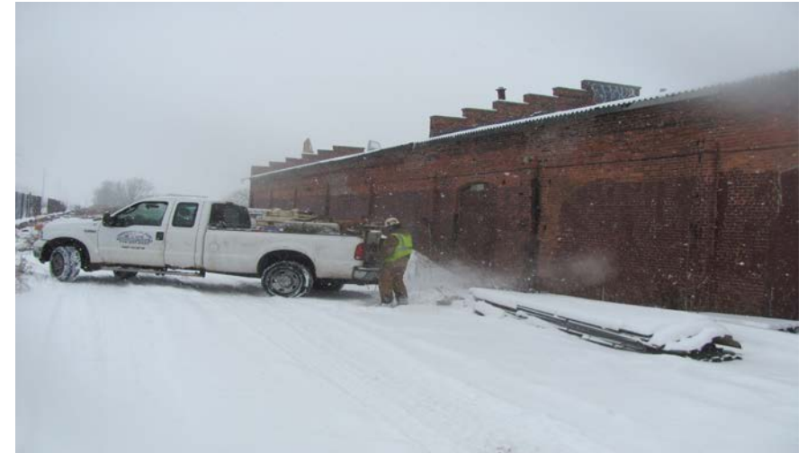
20. Location of Borehole RI-7 facing north-northeast
