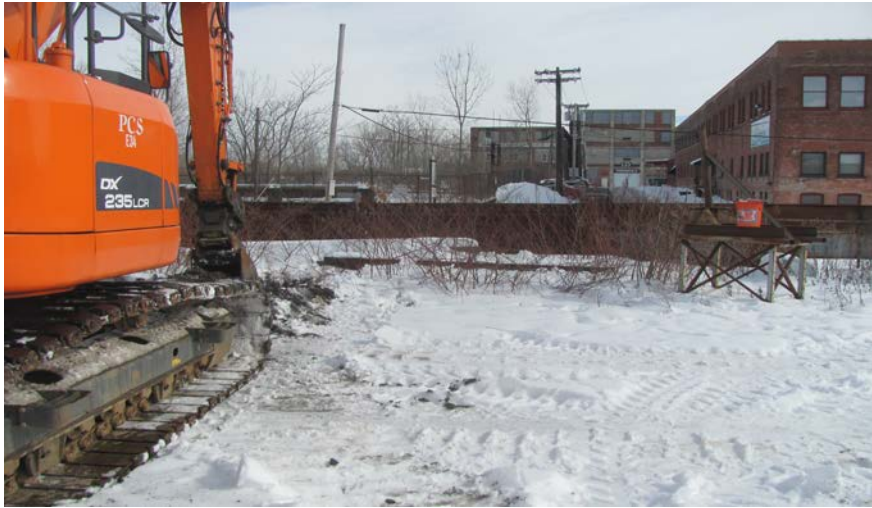
57. Location TP-2 facing east
