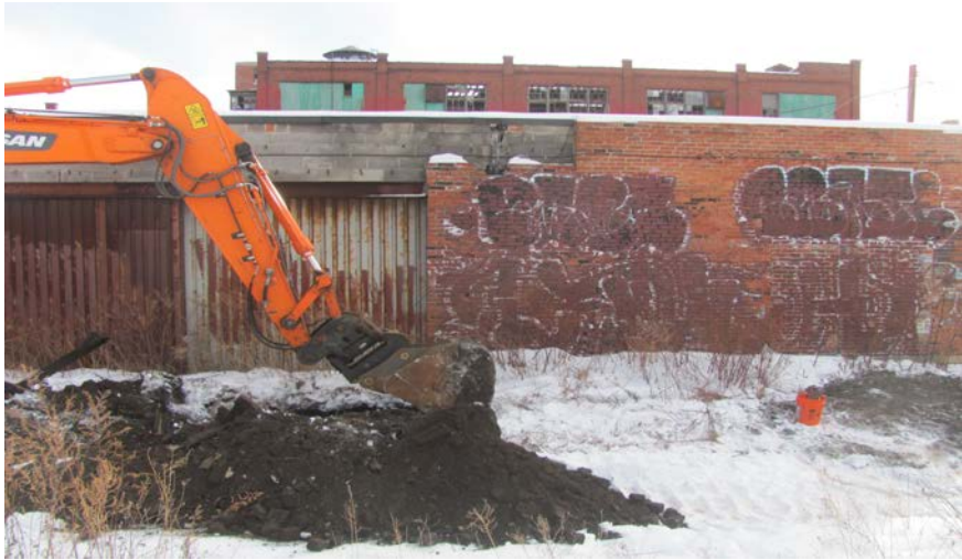
45. Location of Test Pit – TP-5 facing east
