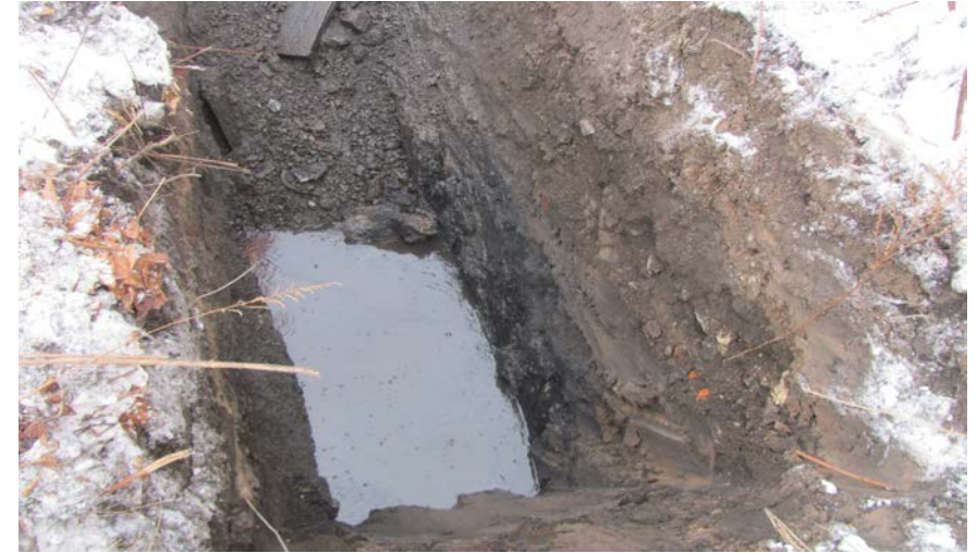
50. View of completed TP-6
