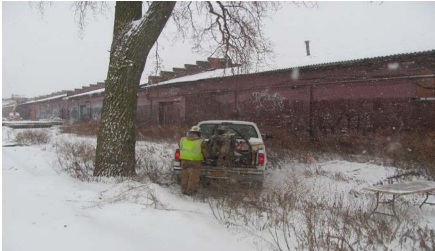
11. Location of borehole RI-4 facing north-northeast
