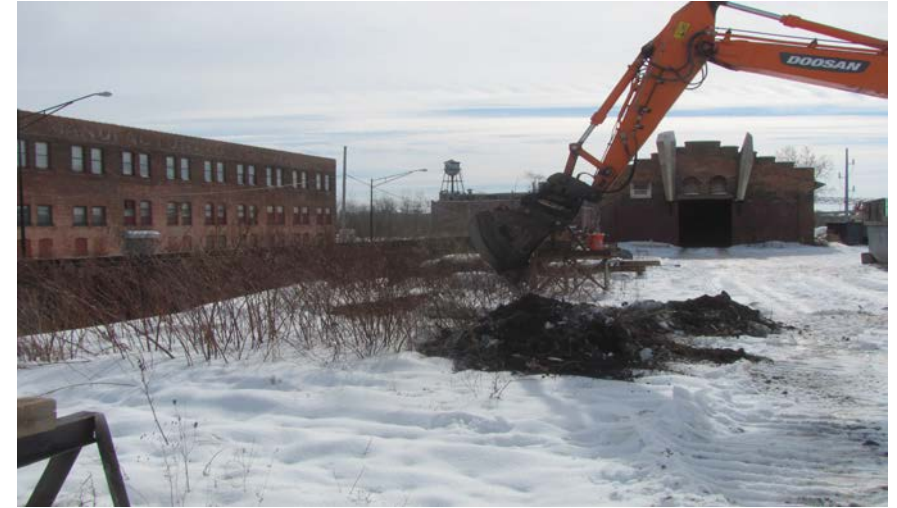
58. View of TP-2 facing south
