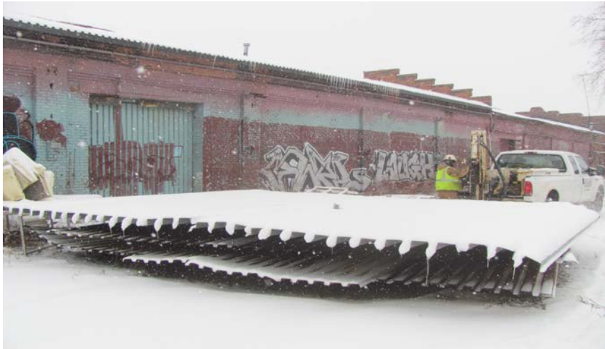
15. Location of Boring RI-5 facing south-southeast
