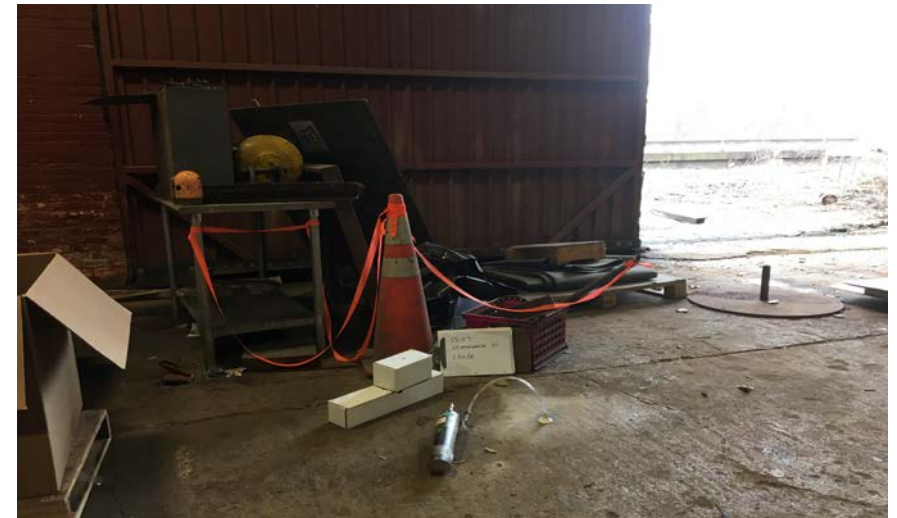
68. SS-03 location facing west
