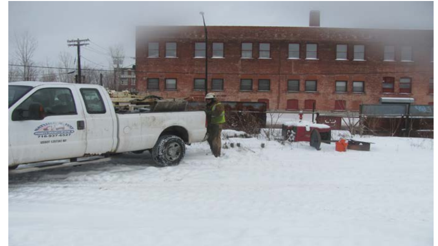
28. Location of borehole RI-10 facing east
