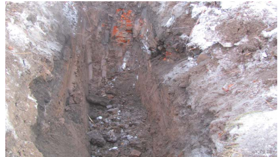
44. View of completed TP-4
