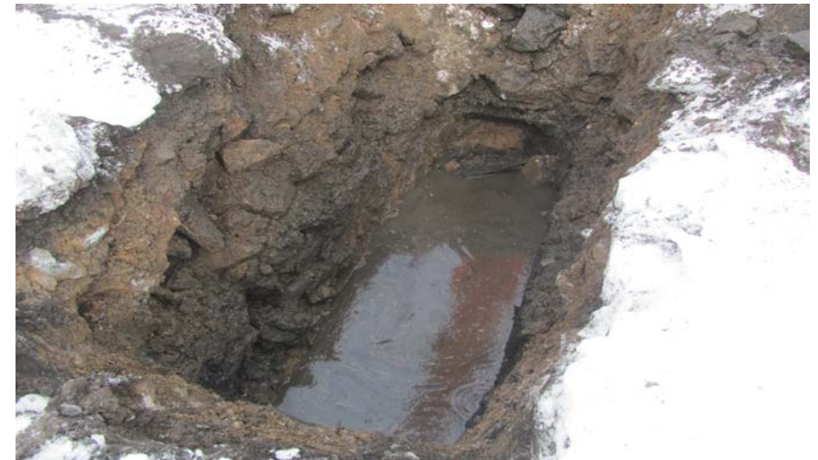
56. View of completed TP-1
