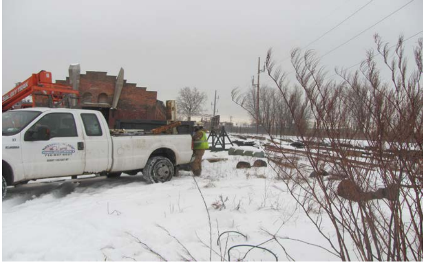
37. Location of borehole RI-13 facing south
