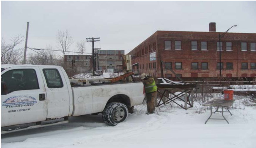
31. Location of Borehole RI-11 facing east
