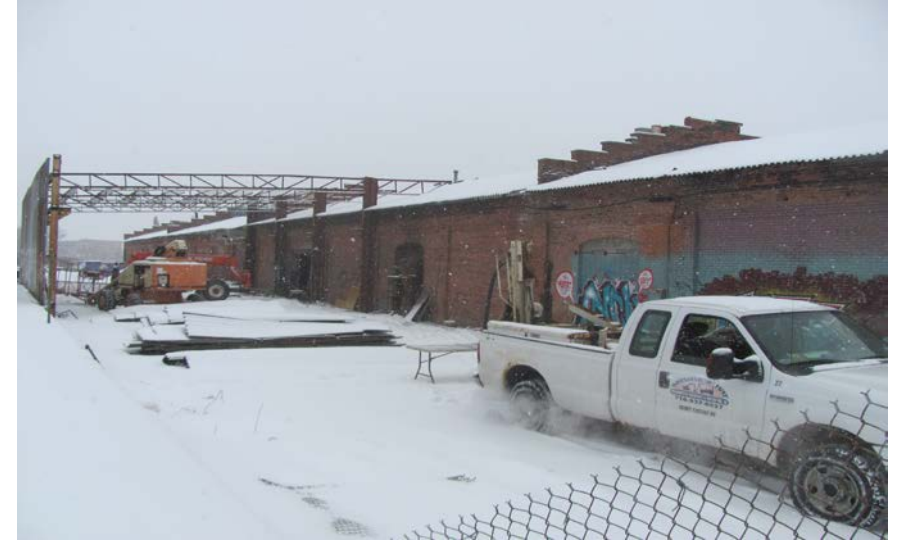
18. Location of Boring RI-6 facing north-northeast
