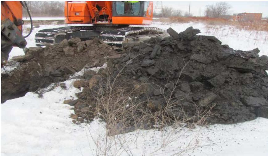
55. View of TP-1 excavated material; wood, brick and pieces of concrete
