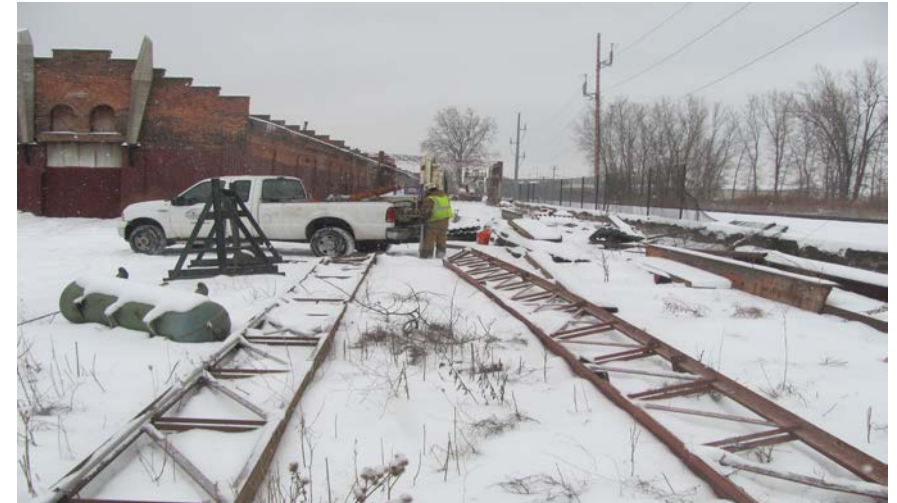
40. View of borehole RI-14 facing south
