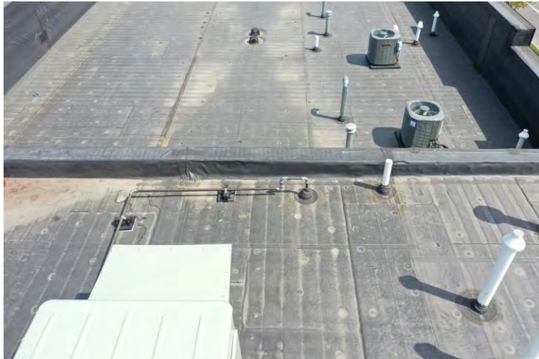
27. Passive SSDS riser #1 located on roof of the commercial side (Hatchet and Hops) of 68 Tonawanda.
