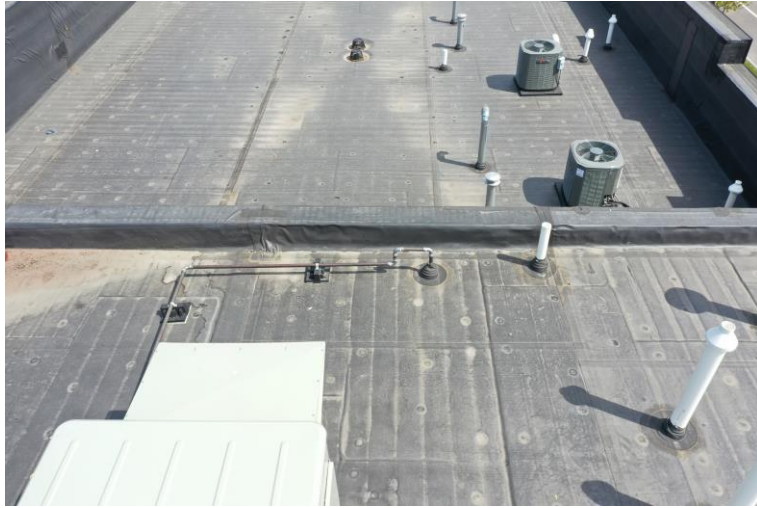
25. Passive SSDS risers located on roof of the commercial side (Hatchet and Hops) of 68 Tonawanda.
