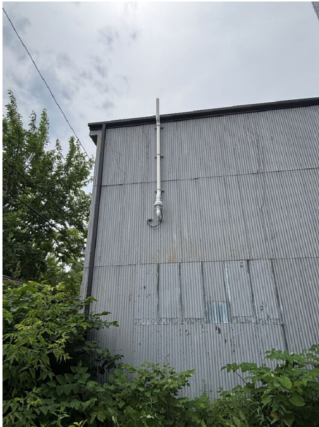
Photograph 5: Exterior exhaust stack with inline fan
