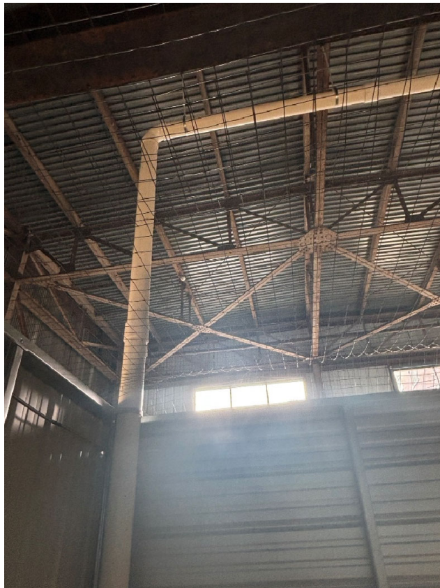
Photograph 2: Riser to north-south horizontal run
