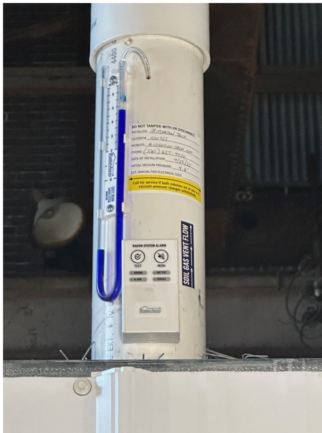
Photograph 6: U-manometer on interior suction point riser
