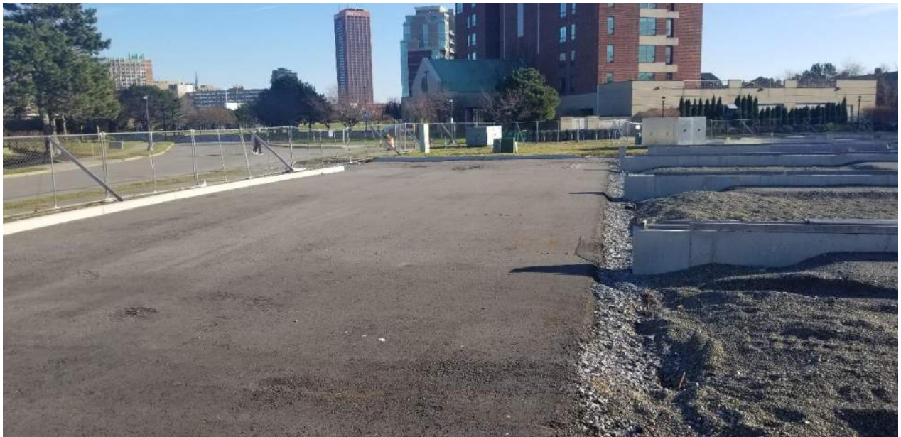
View of Track 4 cover system looking at the corner of Lakefront Boulevard and Ojibwa Circle. Soil Cover Type A and foundations for two future townhome structures.
