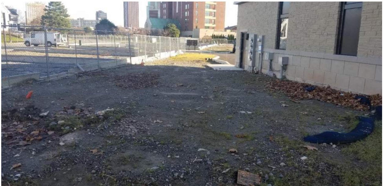
View of the Track 4 cover –landscape areas (Soil Cover Type B) on the east side of the building. Poor grass growth.
