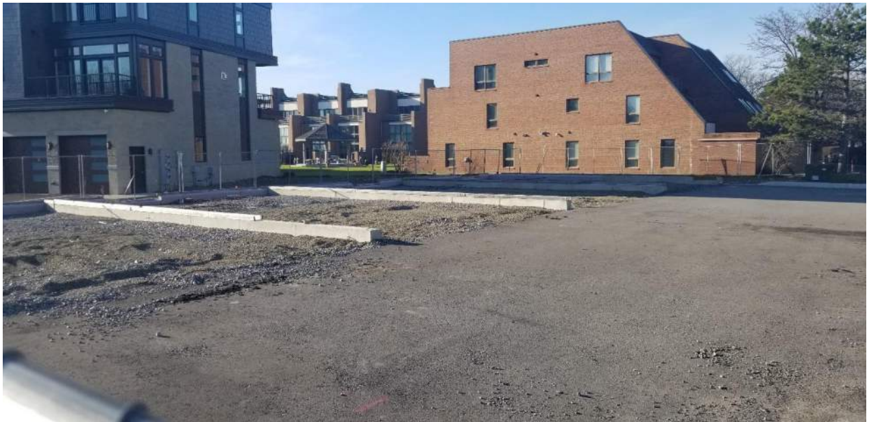
View of the Track 4 cover and foundations for future townhome adjacent to the completed townhome complex (Soil Cover Type A).
