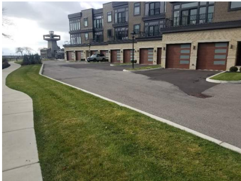
View of the Track 4 cover consisting of eight-unit townhome (Soil Cover Type A) and landscape areas (Soil Cover Type B).
