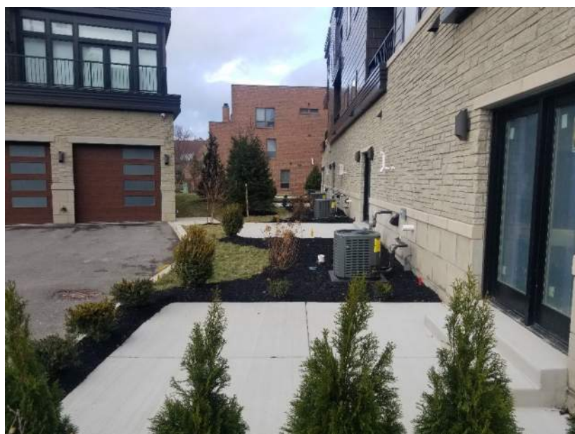
View of Track 4 cover system behind Building A. Soil Cover Type A (building foundations and concrete pad) and landscaped areas.
