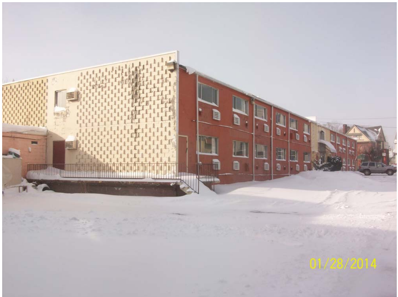
Photo 4: Motel building on the south half of the property looking west toward Main Street.
