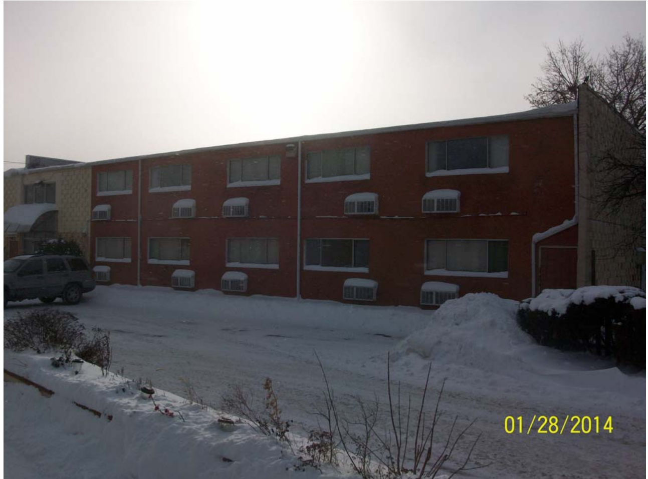
Photo 10: Front (north) side of the motel building located on the south half of the property.
