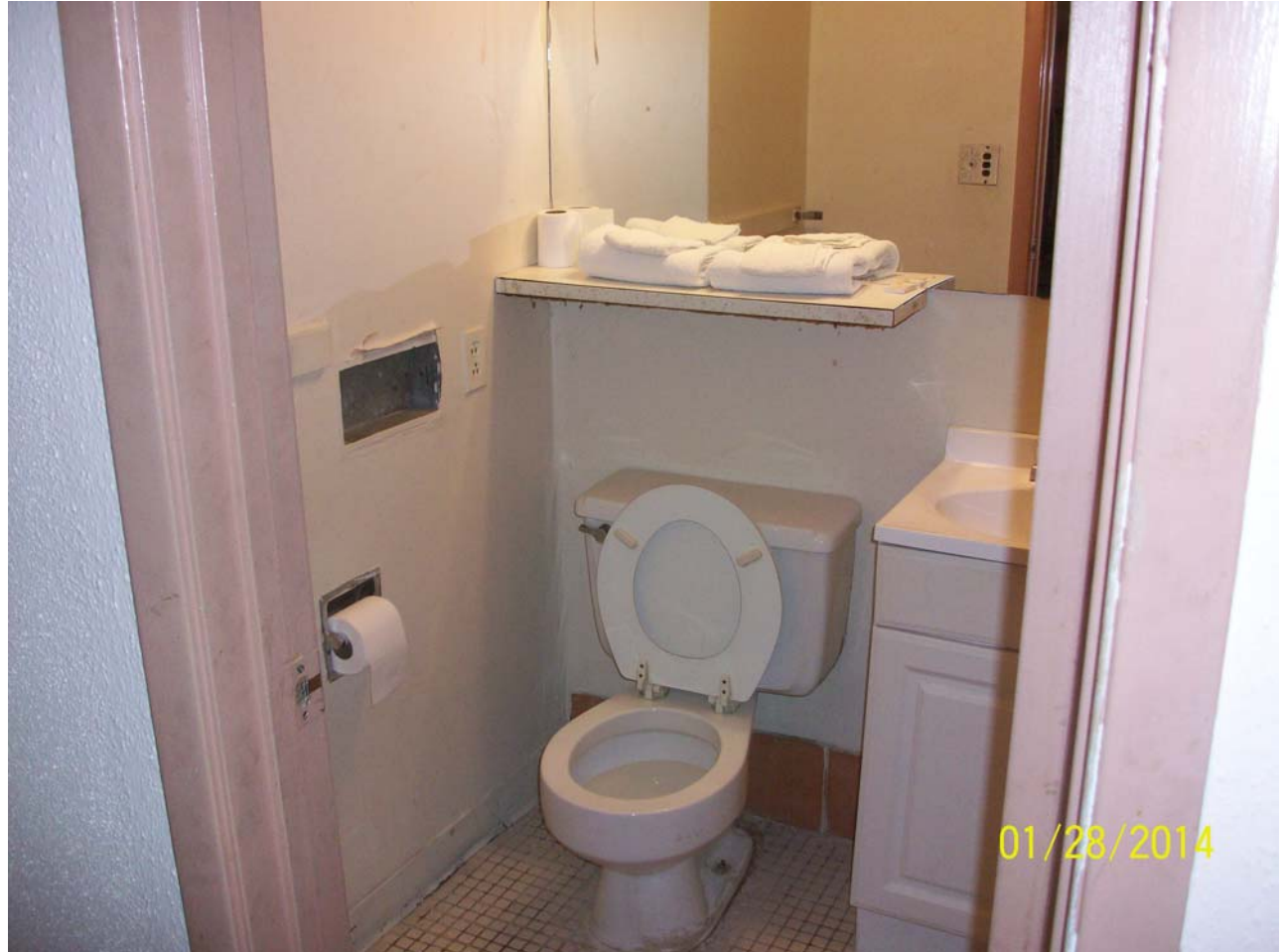
Photo 12: Typical interior conditions of the restrooms in the motel rooms.
