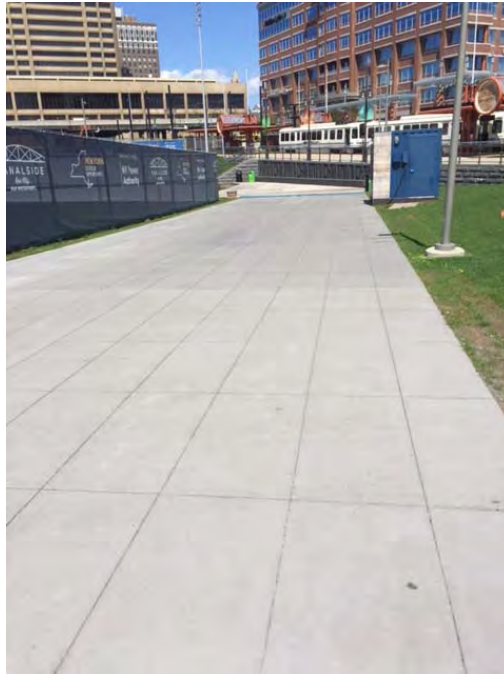
View of the concrete sidewalk along the easterly portion of the Site.
