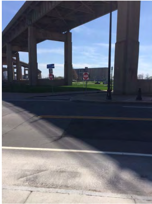
View of the south adjacent park area and the Skyway.
