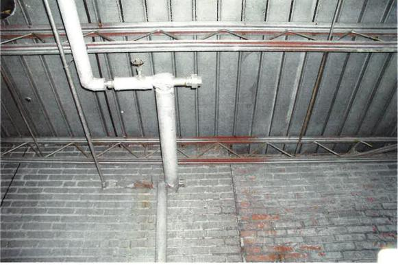
Photograph 16. Potential asbestos containing pipewrap.
