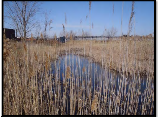
Photo 2: Facing west. Depicts Stormwater Pond 2.
