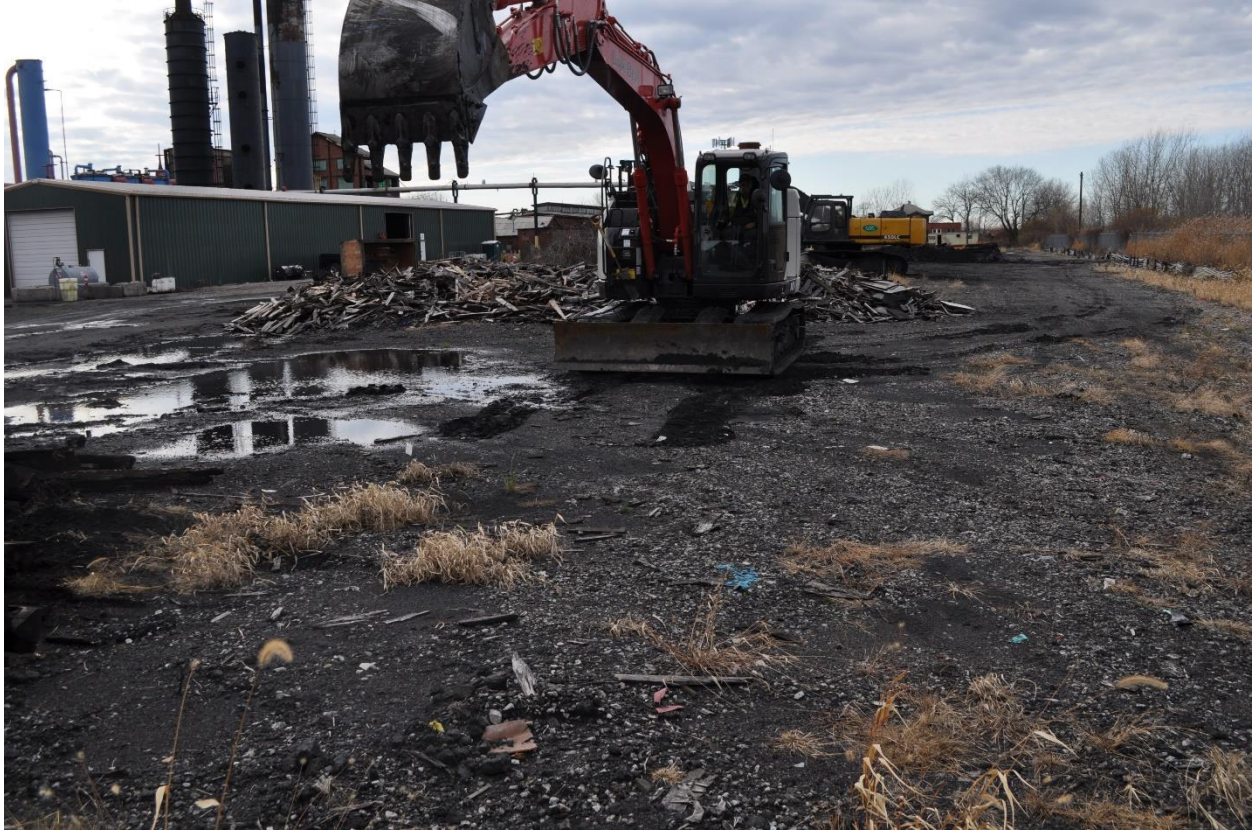
TP-BCP-05 Location Looking West
