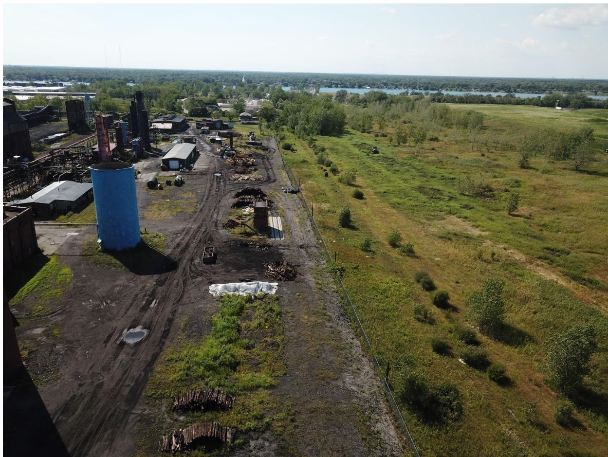
TP-BCP-14 Location Looking West
