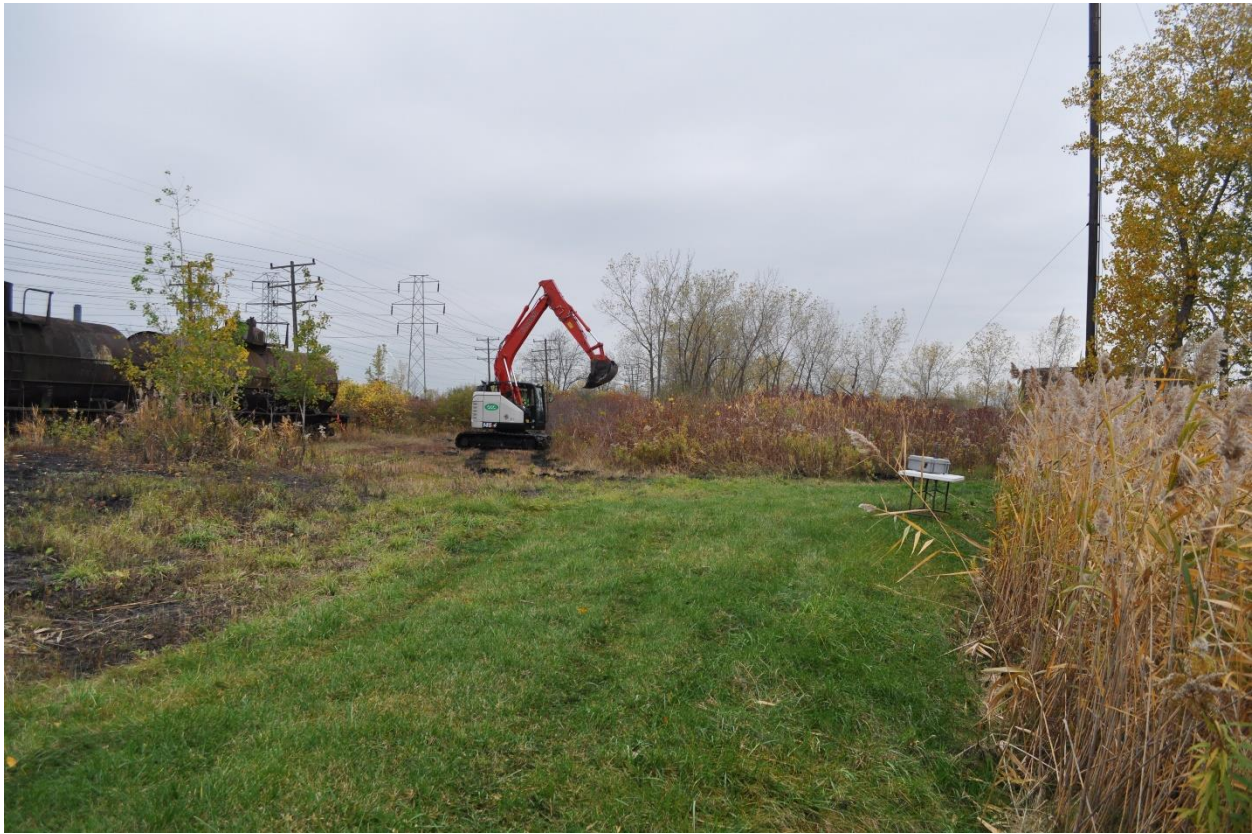
TP-BCP-31 Location Looking West Southwest.
