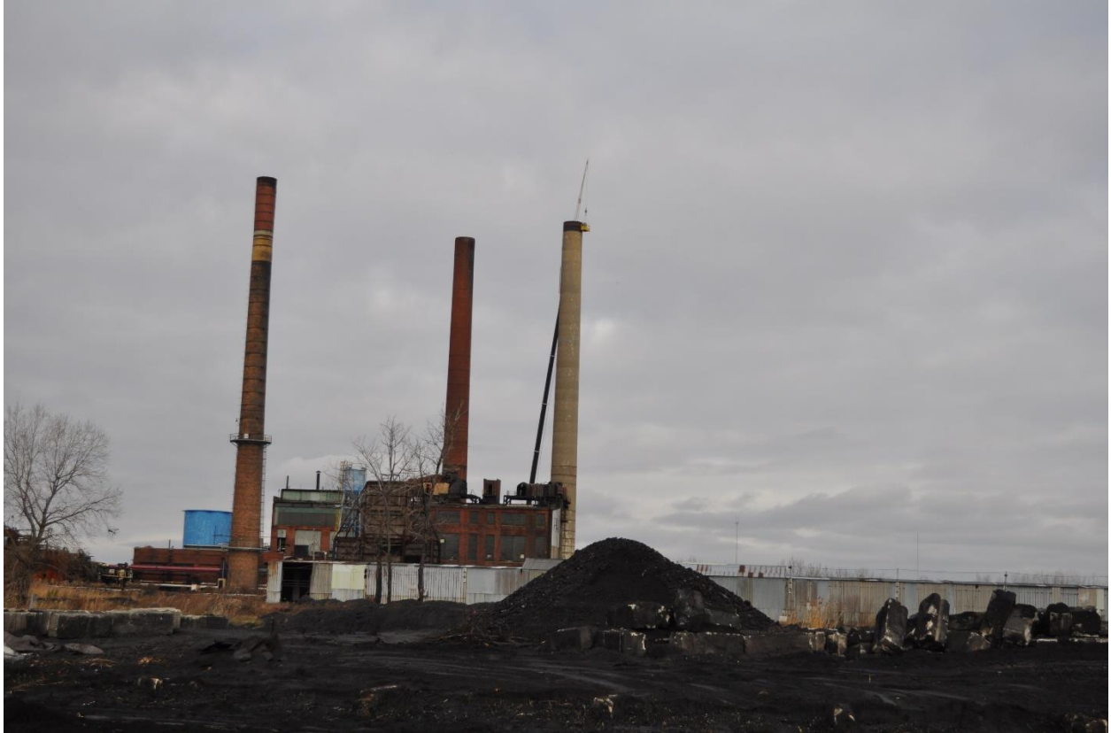
TP-BCP-30 Location Looking North
