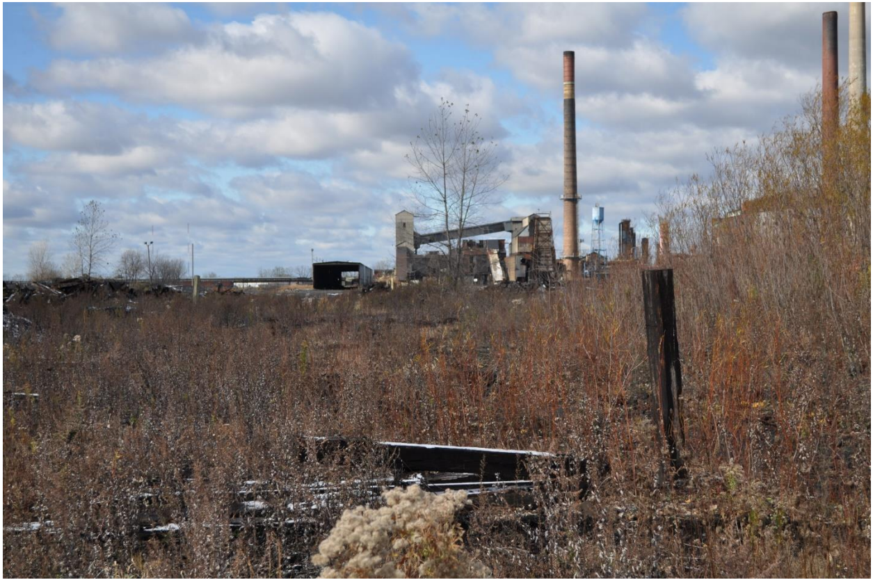
North end of TP-BCP-09 Location Looking West
