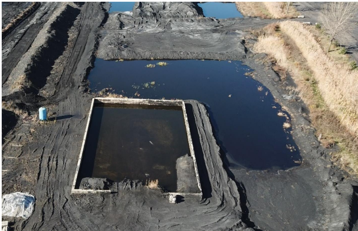
TP-BCP-23 Location Looking West
