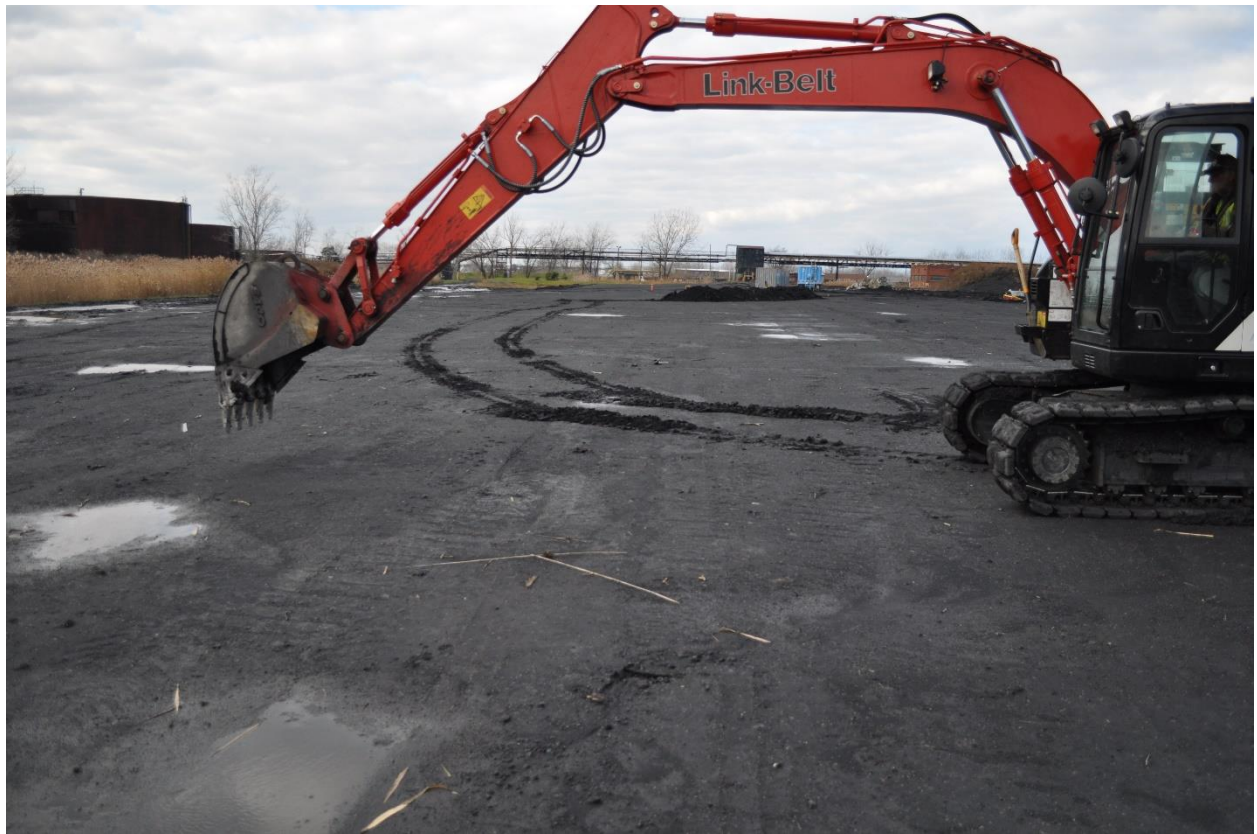
TP-BCP-29 Location Looking West
