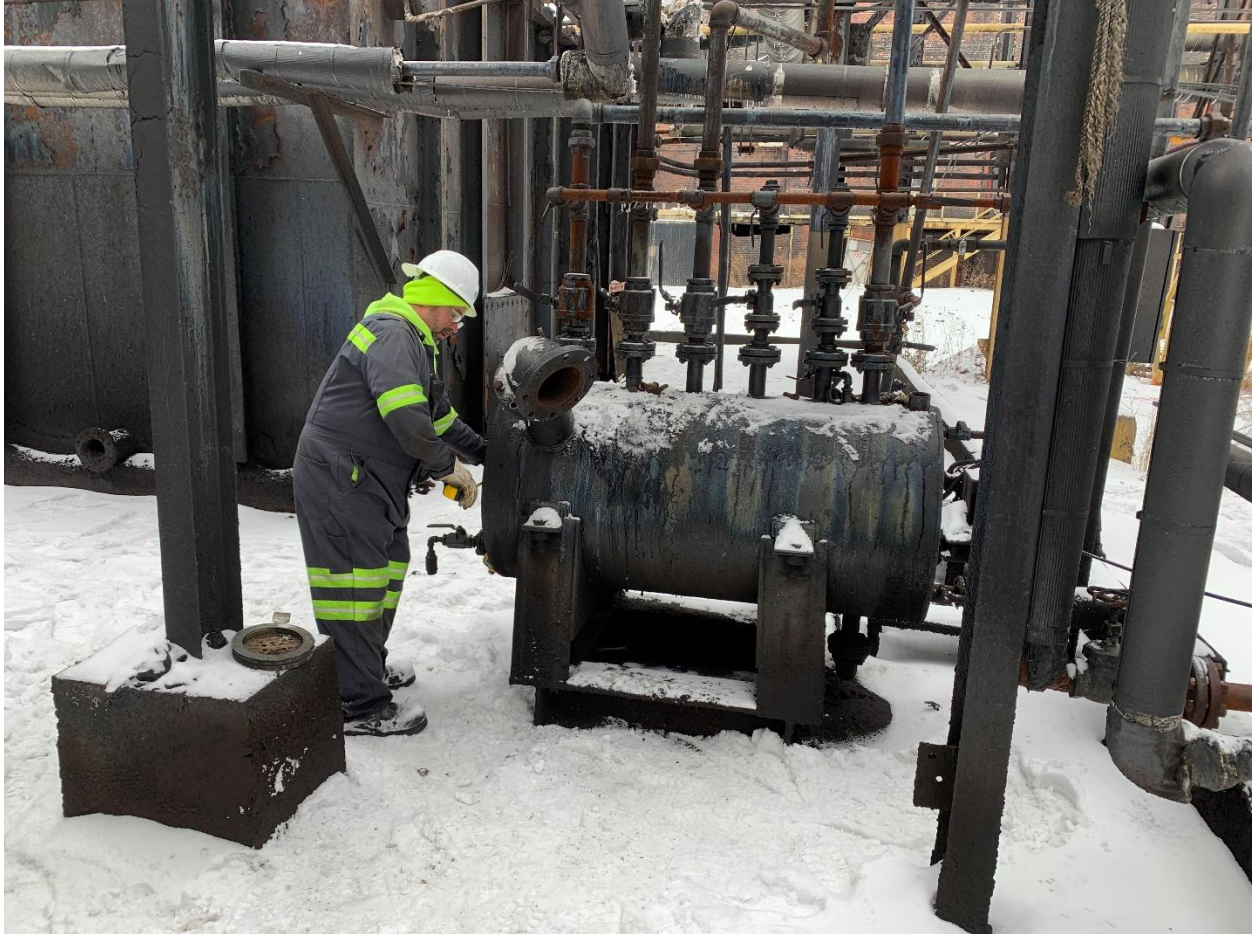
Photograph No. 2: The former flow through dehydrator tank PT15.
