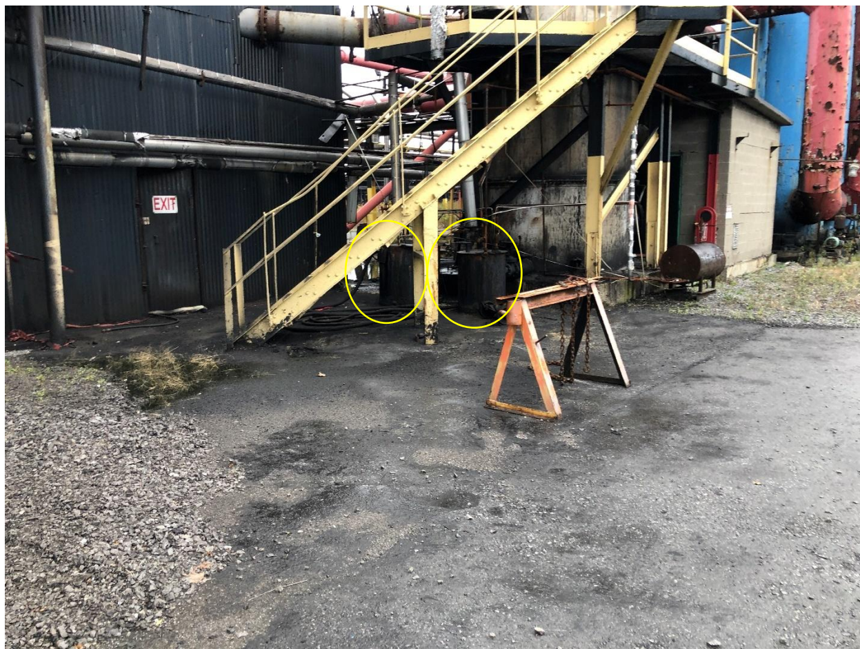
Photograph No. 1: Location of presumed tanks ST25 and ST26.
