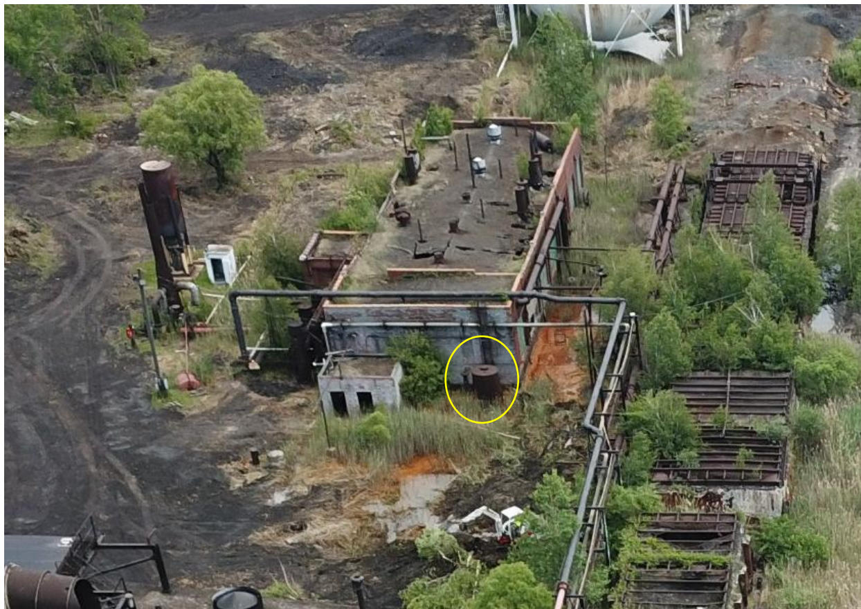
Photograph 4: ST28 was located on the southwest corner of the former compressor building.
