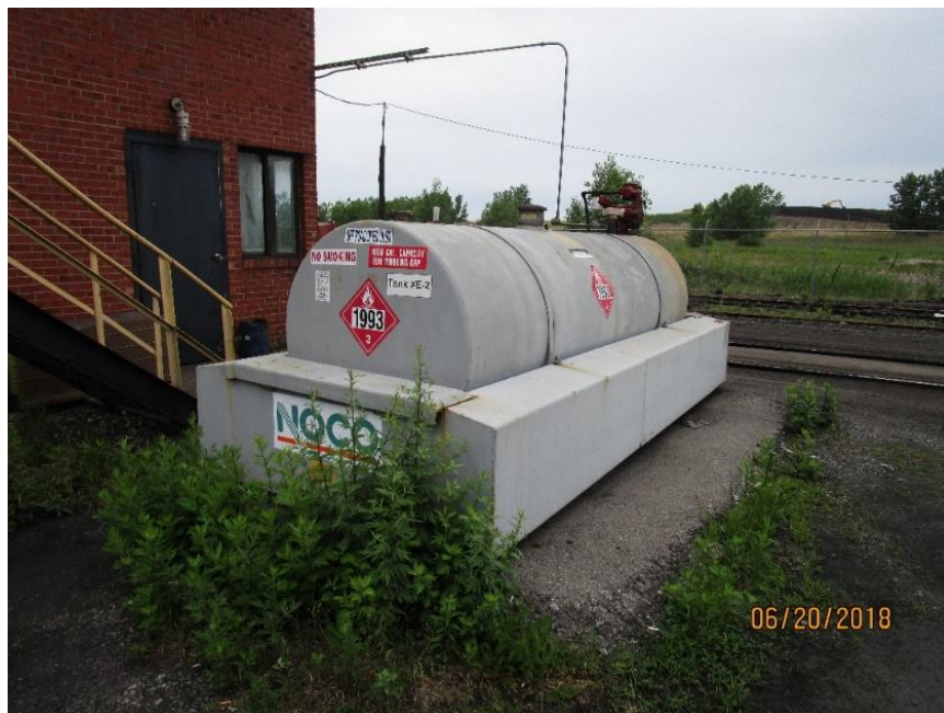
Photograph No. 1: PBS tank E02, just east of the former Rail Scale Building (Grid Location Y2).
