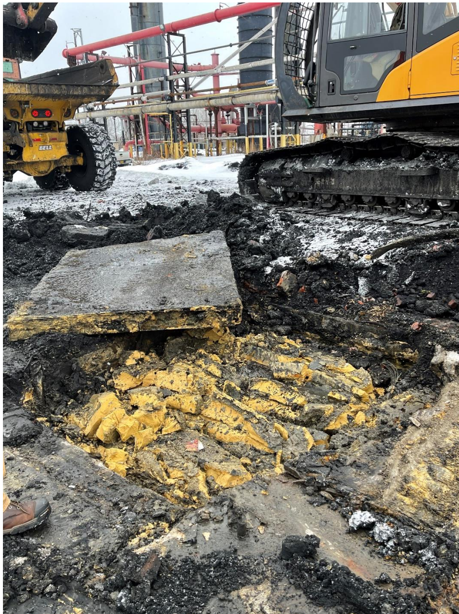
Photograph 4 – Lid Seal in Former Elevator Shaft
