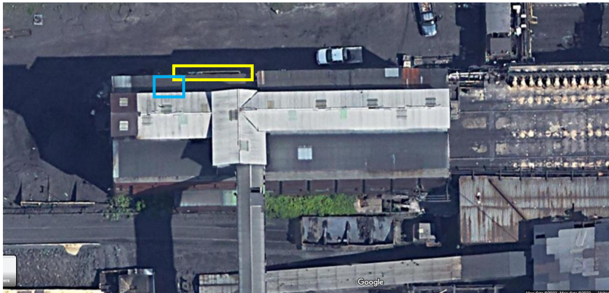
Photograph 1: Aerial view of the former Coal Charging Building.
