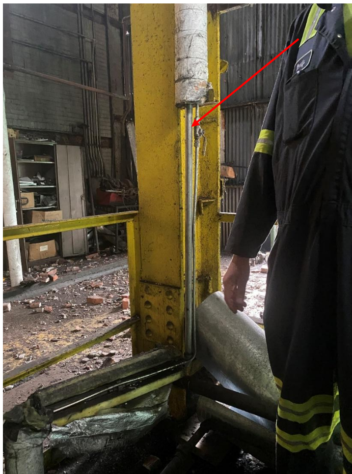
Photograph No. 3: Chemical Feed Tubing on Production Floor of the former Boiler House
