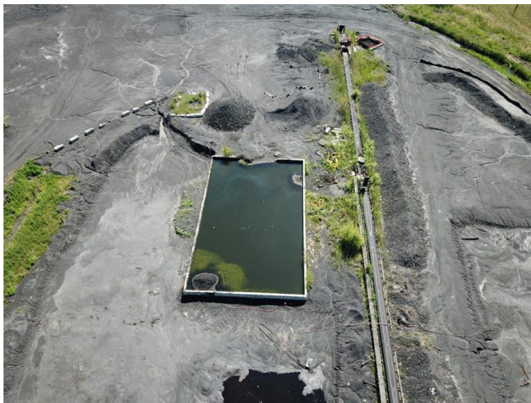
Mixing Pad, June 18, 2020 View Looking Down and Toward the East
