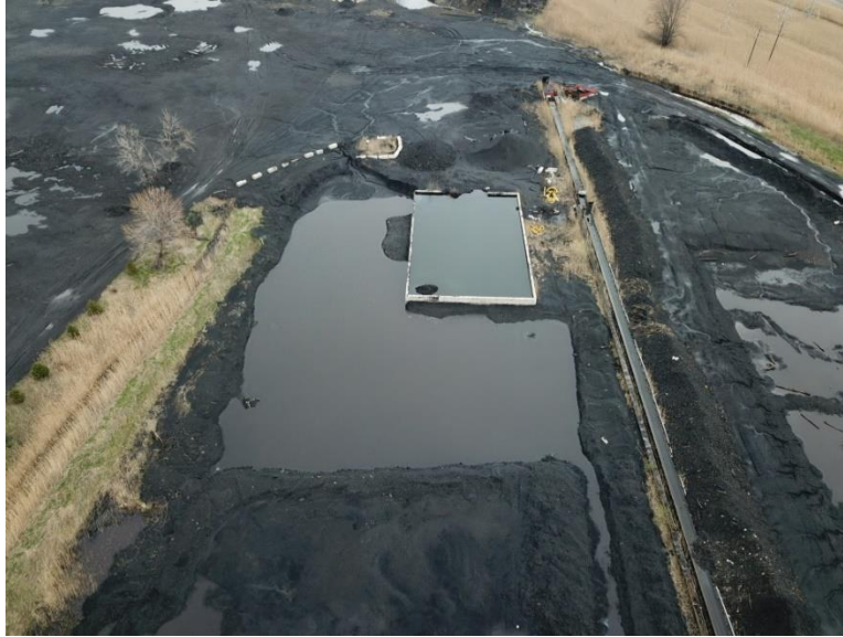
Mixing Pad, May 2020 View Looking Down and toward the East
