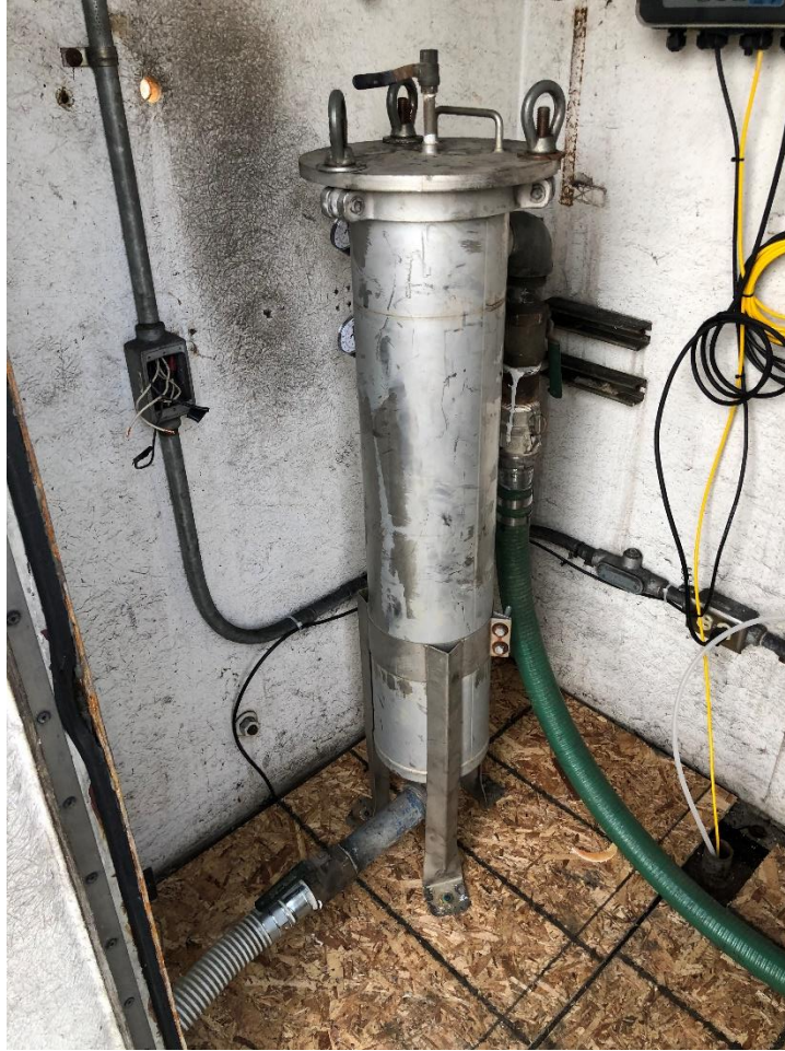
Secondary – 10 Micron Bag Filter December 2020
