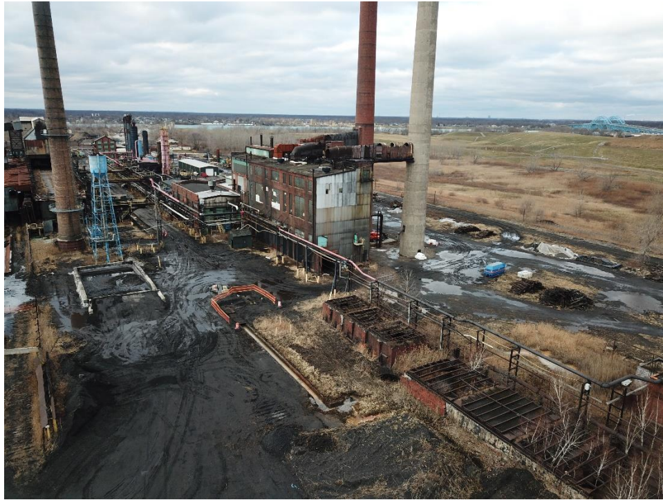
Box Culvert Cleaning – East End December 2020
