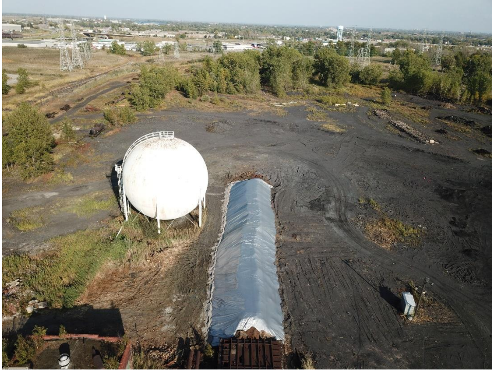
Iron Oxide Piles Protected from Weather October 2020
