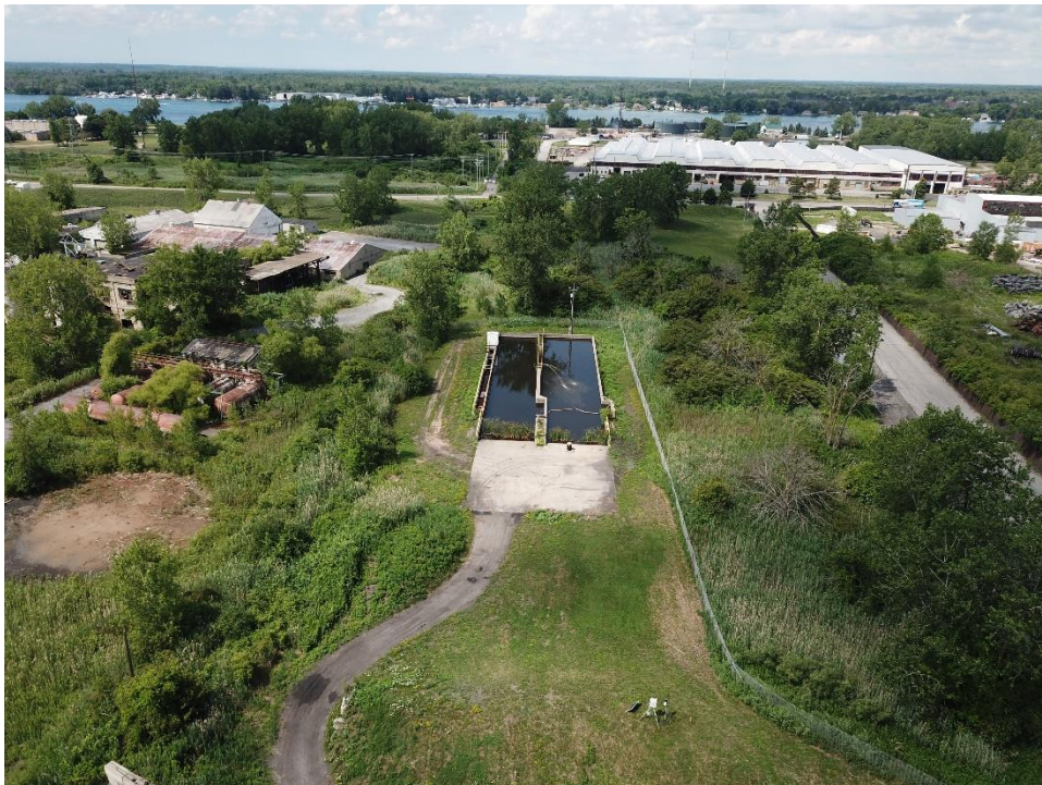
Aeration System – Settling Ponds August 2020
