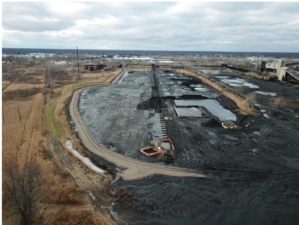
Regraded South Coal Yard and South Ditch Road Improvements December 2020
