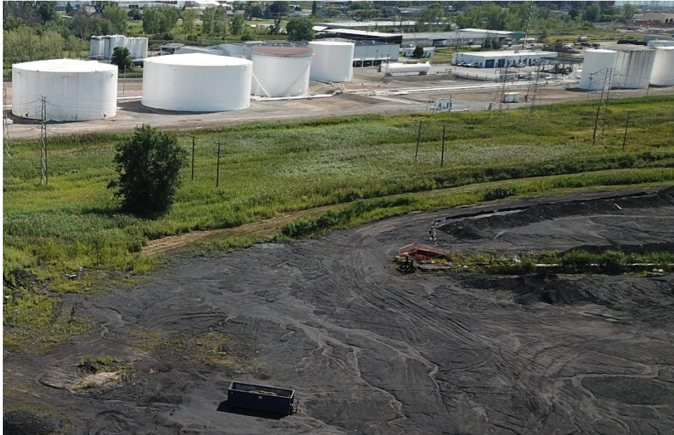
East End of South Drainage, with Check Dams August 2020
