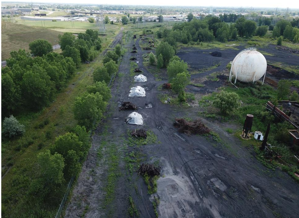
Soil Piles Left by Others – Protected from Weather October 2020
