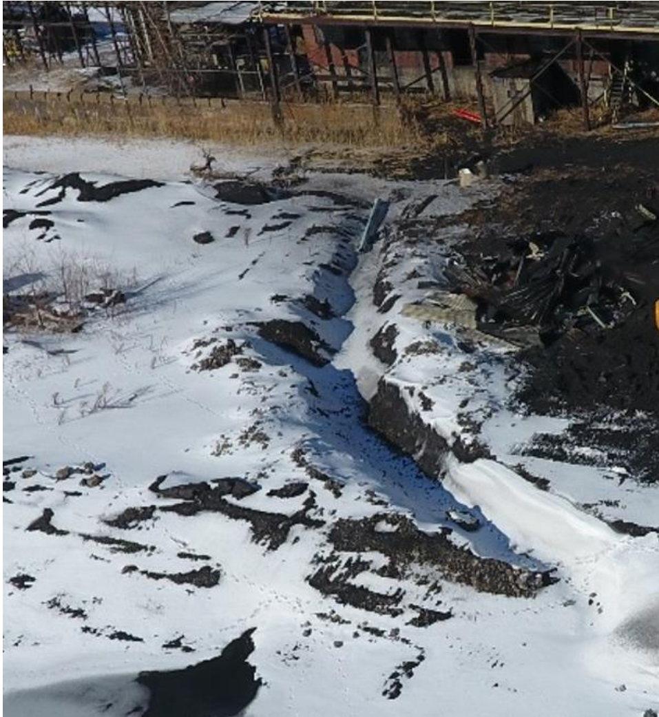
Photograph No. 3 Drainage Features to be Filled
