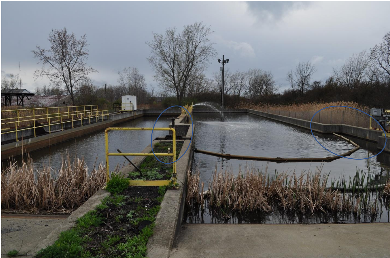
Sediment Traps in Settling Ponds
