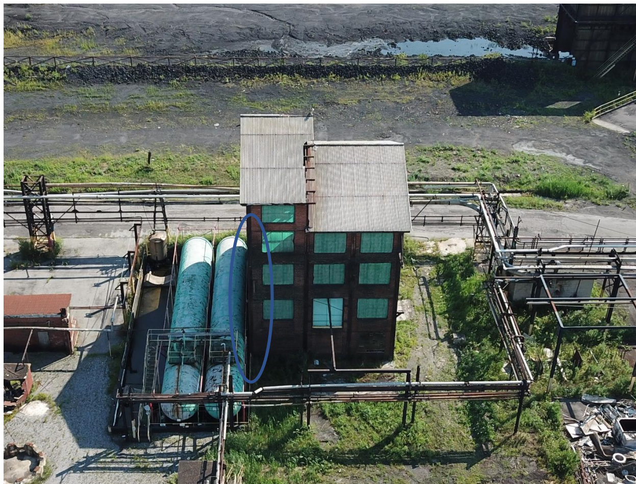
Photograph No. 1 - Common Wall between Secondary Containment and Former Light Oil Building.
