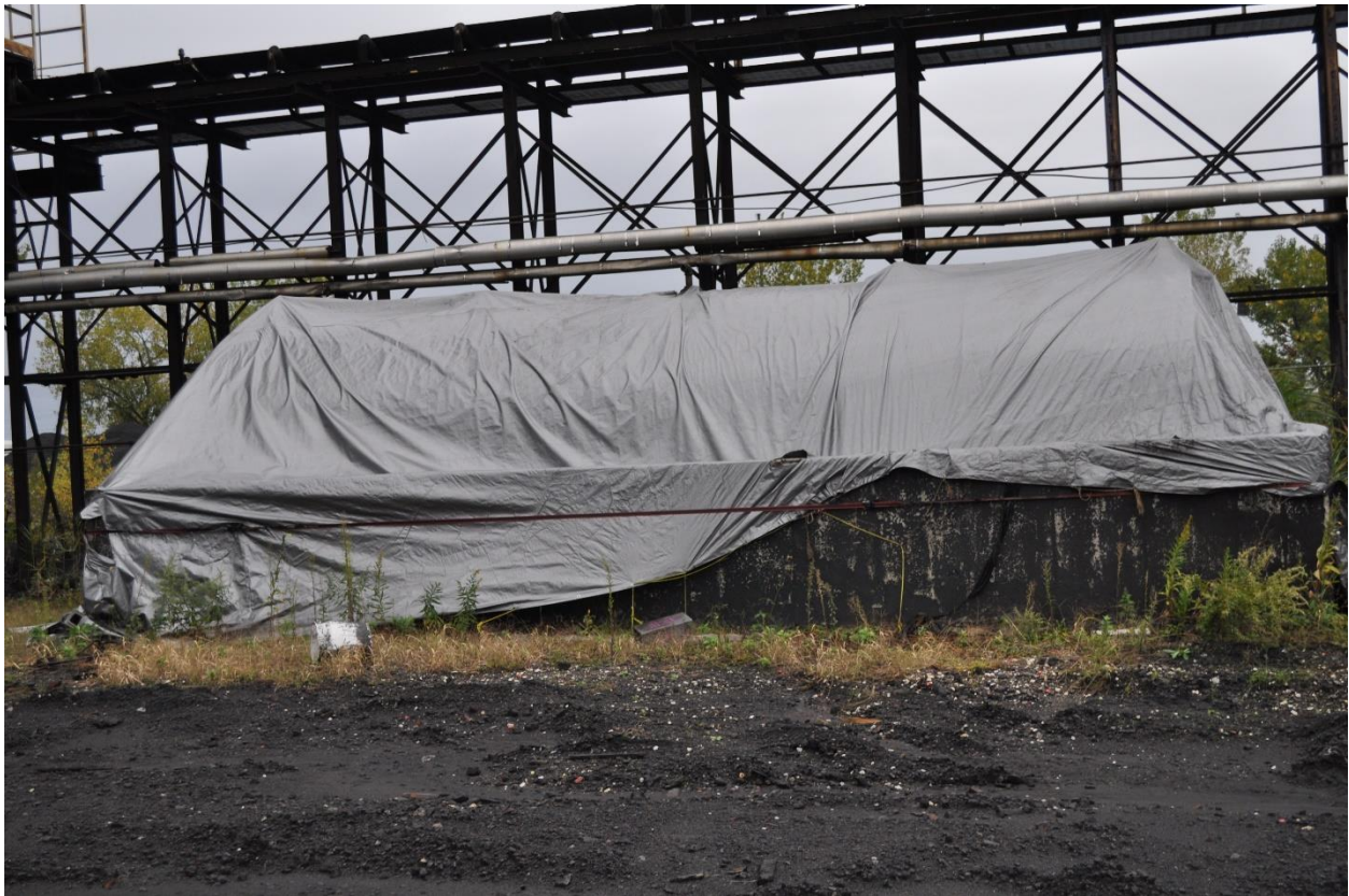
Reinforced Concrete Secondary Containment Around Waste Oil Tank
