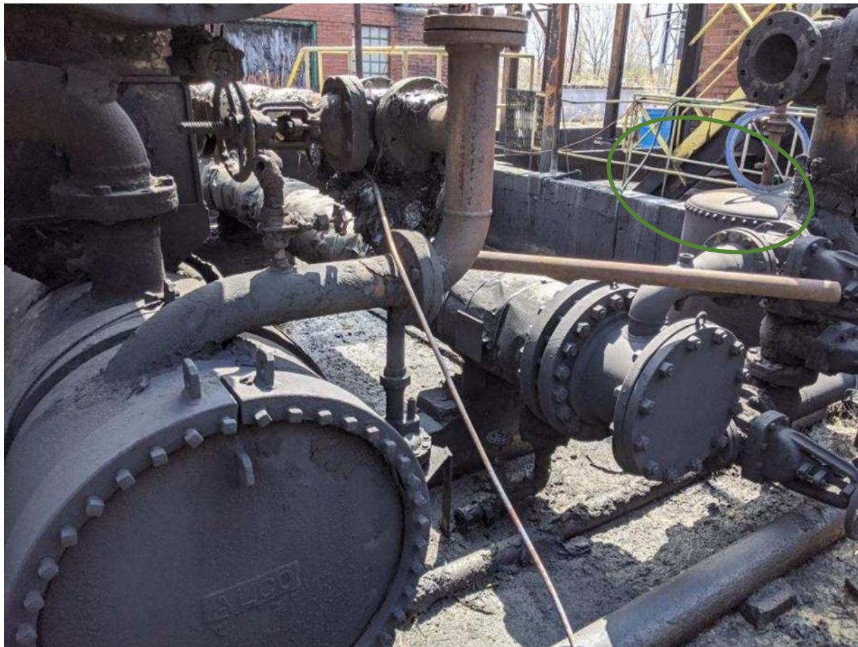
Photograph No. 3 – Shared Wall in Light Oil Area
