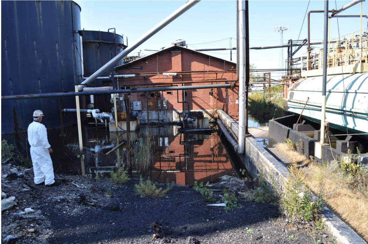
Photograph No. 5 - Separation between Weak Ammonia Secondary Containment and the Light Oil Area Secondary Containment
