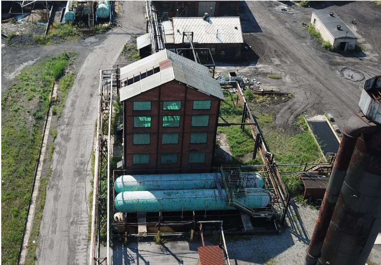
Former Light Oil Area Tanks and Secondary Containment
