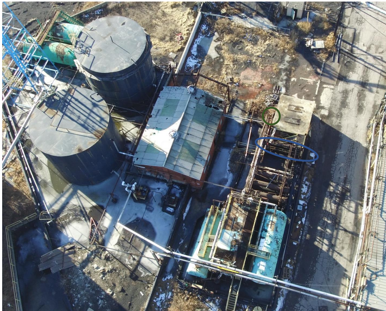
Photograph No. 2 - Secondary Containment for Light Oil Area Tanks PT04, PT12 and PT13
