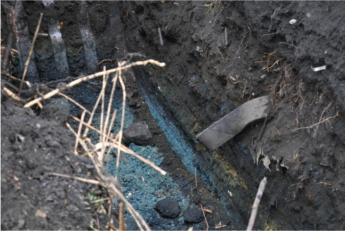
Photograph 1: TP-BCP-35 – Typical Layer of Blue Stained Fill
