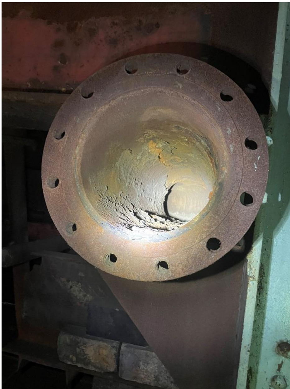
Photograph A-12 10-inch COG pipe where it tied into Boiler/ furnace. Note little scale build-up observed.
