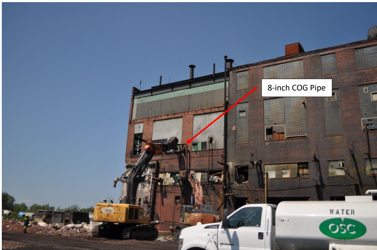
Photograph No. 9 8-inch COG Line on South Wall of the Boiler House
