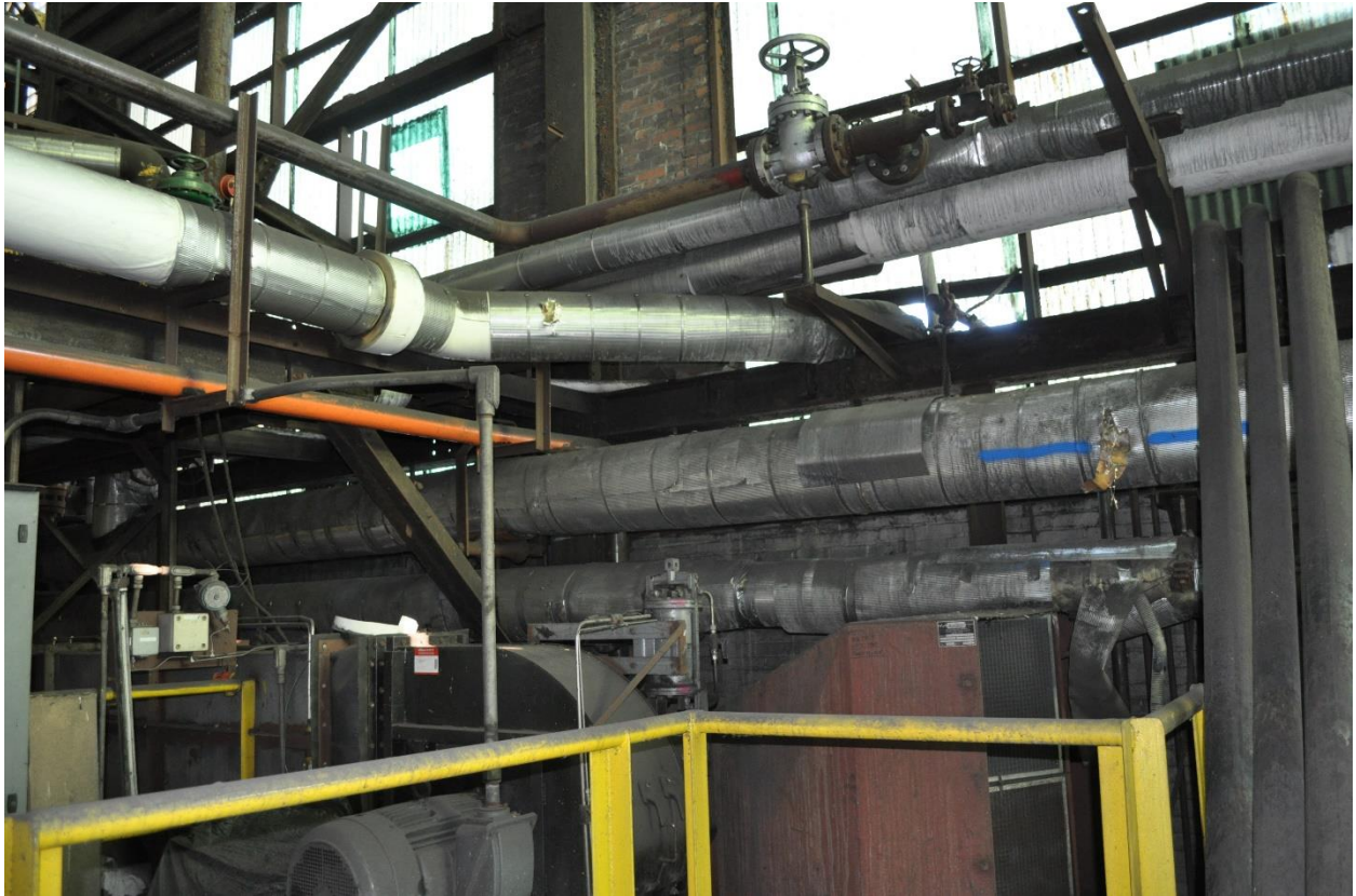
Photograph A-14 Interior Section of 8-inch Pipeline inside the Boiler House
