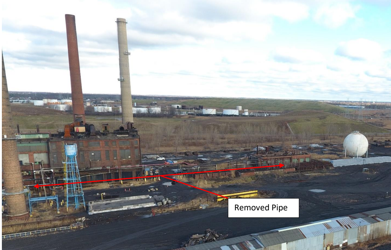
Photographs No. 1 Coke Oven Gas Lines Removed Before Fire
