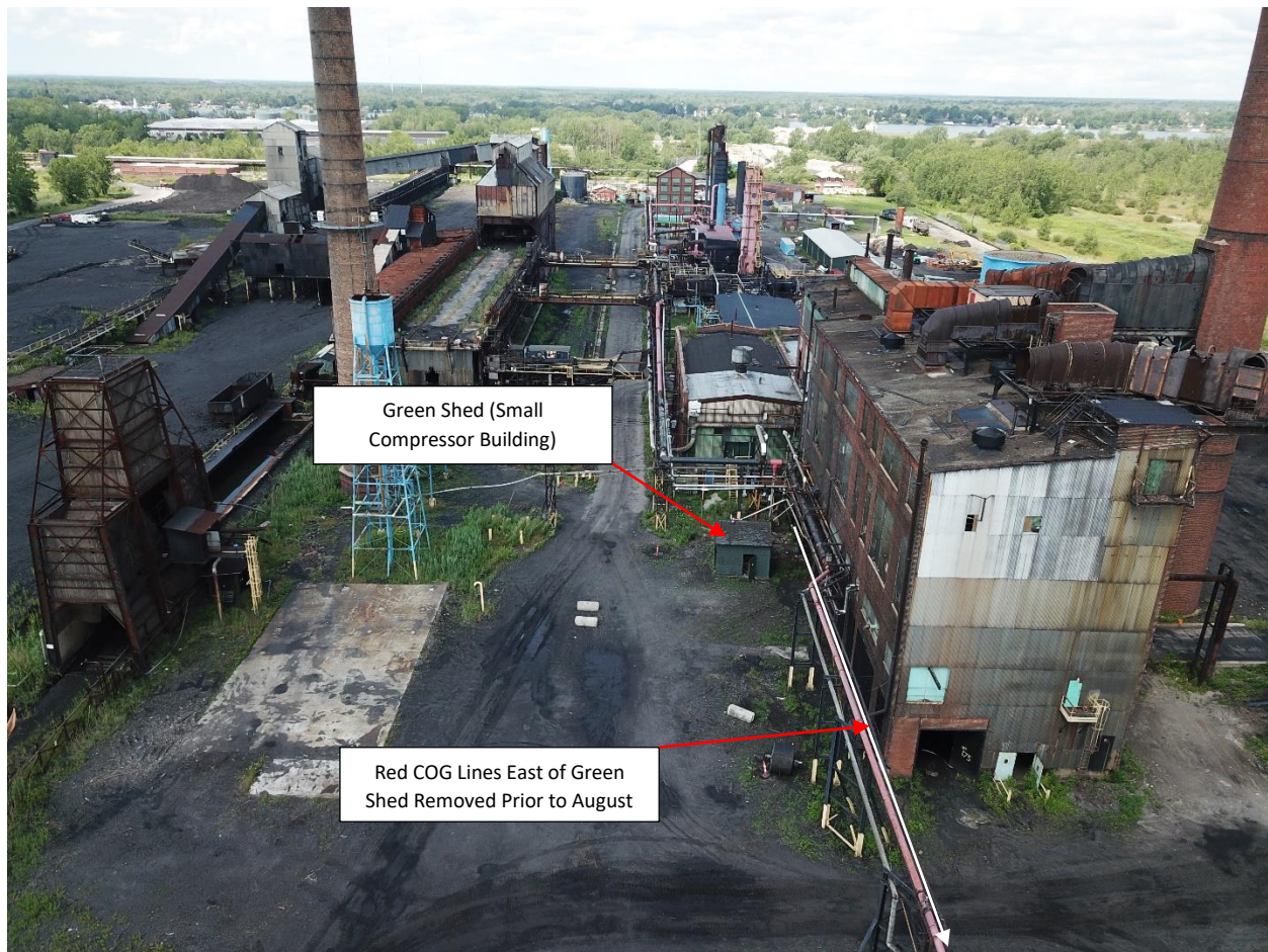
Photograph No. 2 COG pipes Removed Before August 2021 Without Incident
