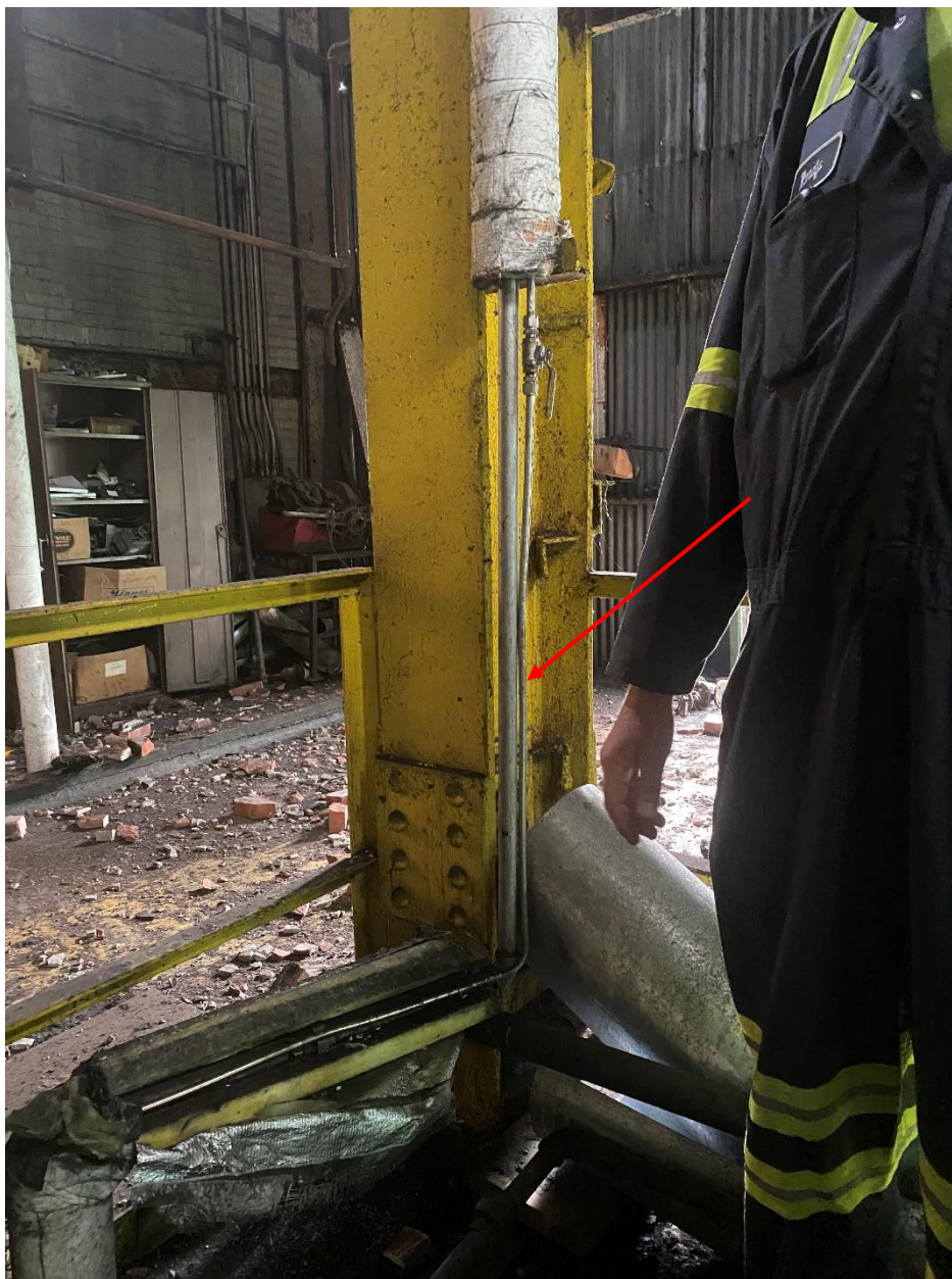
Photograph No. 3: Chemical Feed Tubing
