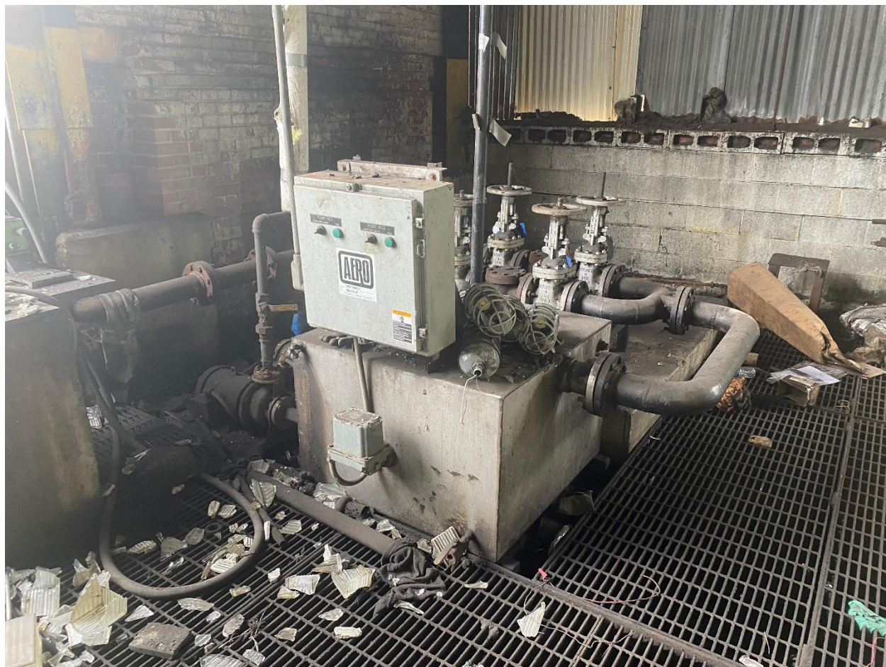
Photograph No. 2: Chemical Feed Pump (Note: This is on the ground floor, one level below the Lime Still)
