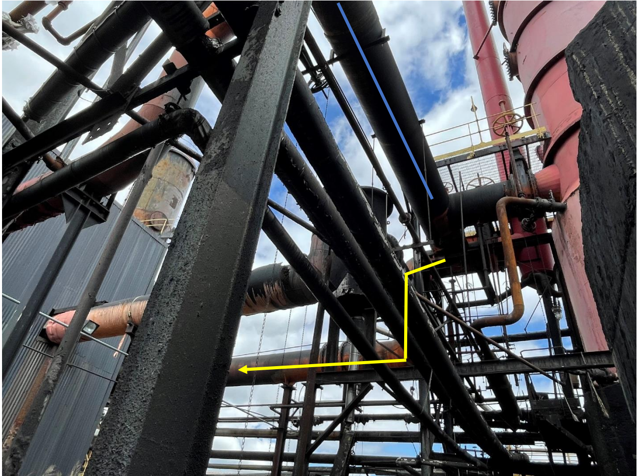
Photograph 5: The blue line is the pipe shown in Photograph 3 to the tar decanter. The yellow line is a 24-inch to 30-inch line from the Primary Cooler to the Secondary Cooler, prior to the Exhausters.
