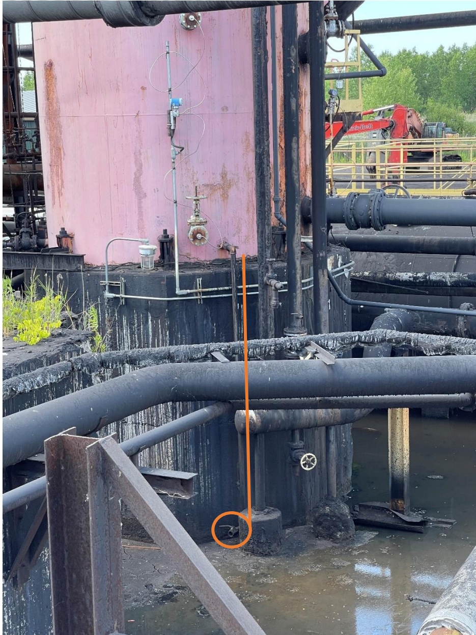
Photograph 8: Small pipe from Cooler base to valve.
