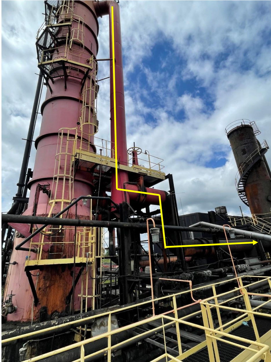
Photograph 6: Line from primary to secondary cooler.
