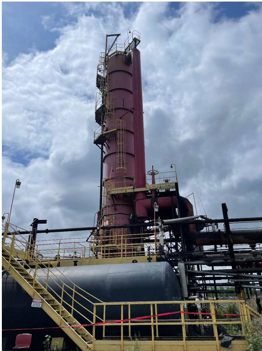
Photograph 1: Primary Cooling Tower, eastern most process vessel, first Coke Oven Gas (COG) process vessel.
