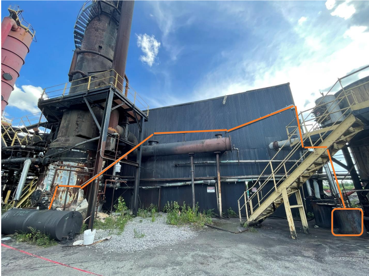
Photograph 10: A 2-inch line from tank north of Secondary cooler to the tar precipitator condensate sump east of Tar Precipitator.
