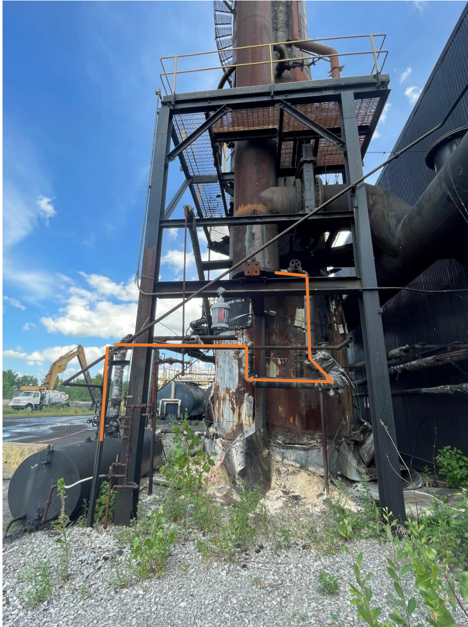
Photograph 11: 2-inch line coming from main vertical drip pod on Secondary Cooler.
