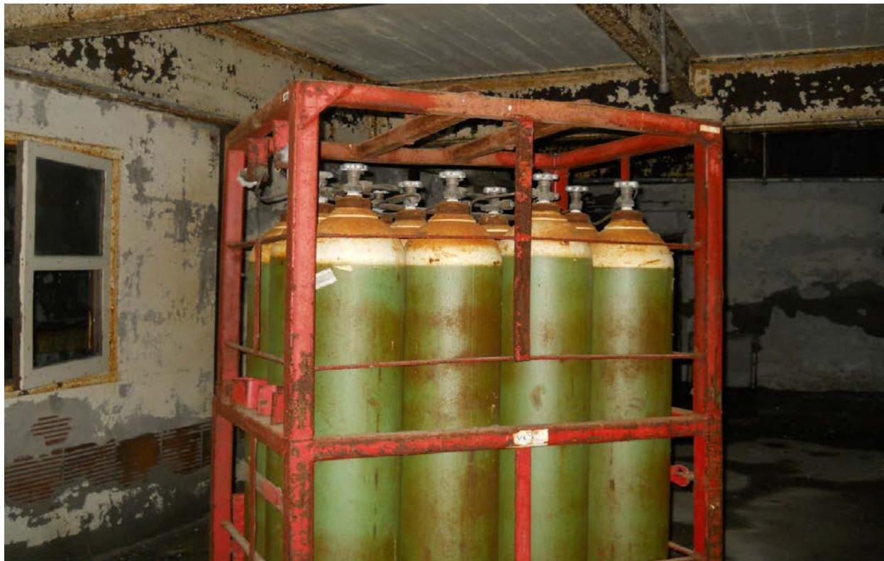
PHOTO #2- Photograph of oxygen cylinders in Building 1.
