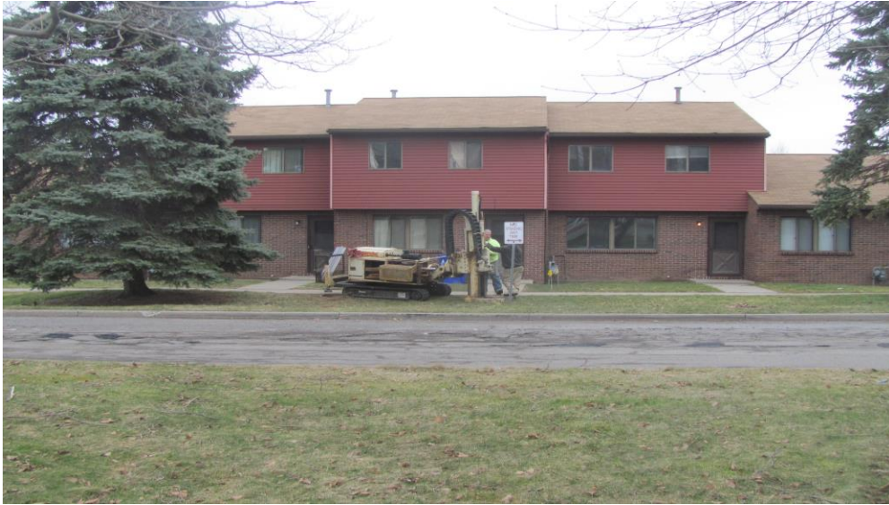
37. Location of Borehole BH-13 from south across Holloway Blvd. facing north
