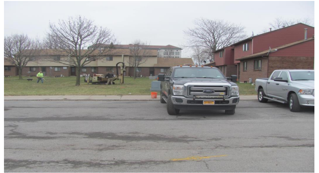
34. Location of Borehole BH-12 from west facing east
