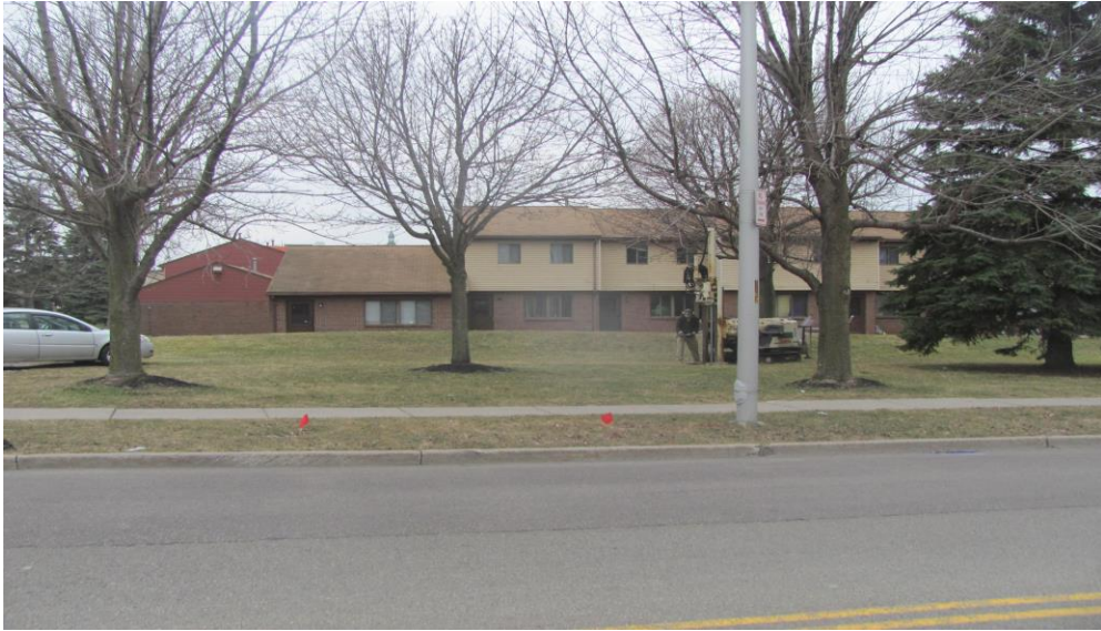
21. Location of Borehole BH-7 east side of Michigan Ave. facing west
