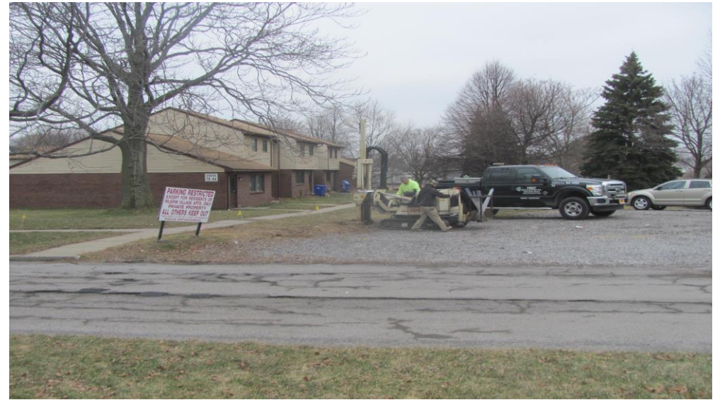
26. Location of Borehole BH-9 from south facing north west
