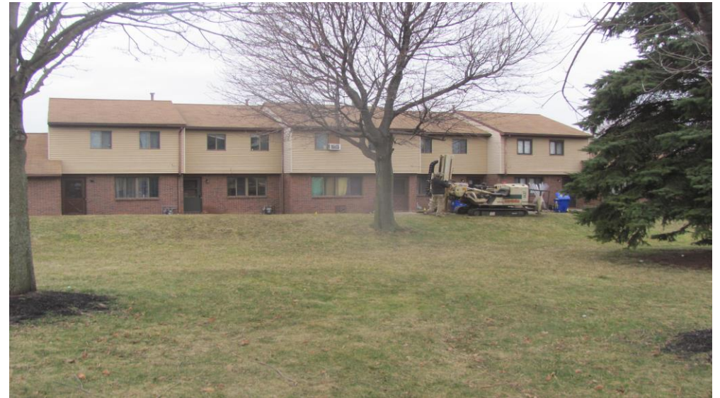
18. Location of Borehole BH-6 from east along Michigan Avenue facing west
