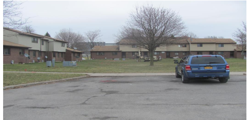
32. Location of borehole BH-11 from west facing east
