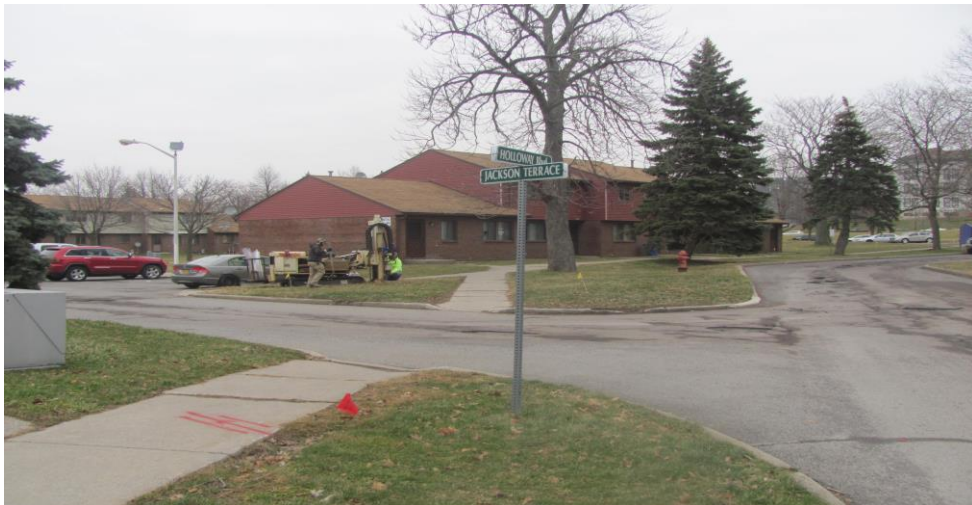
3. Location of BH-1 from southwest facing northeast
