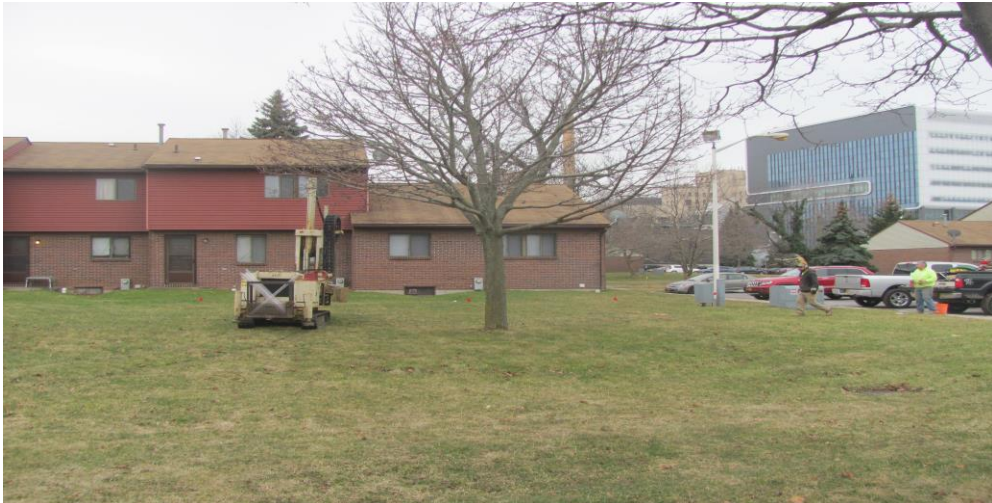
35. Location of Borehole BH-12 from north facing south
