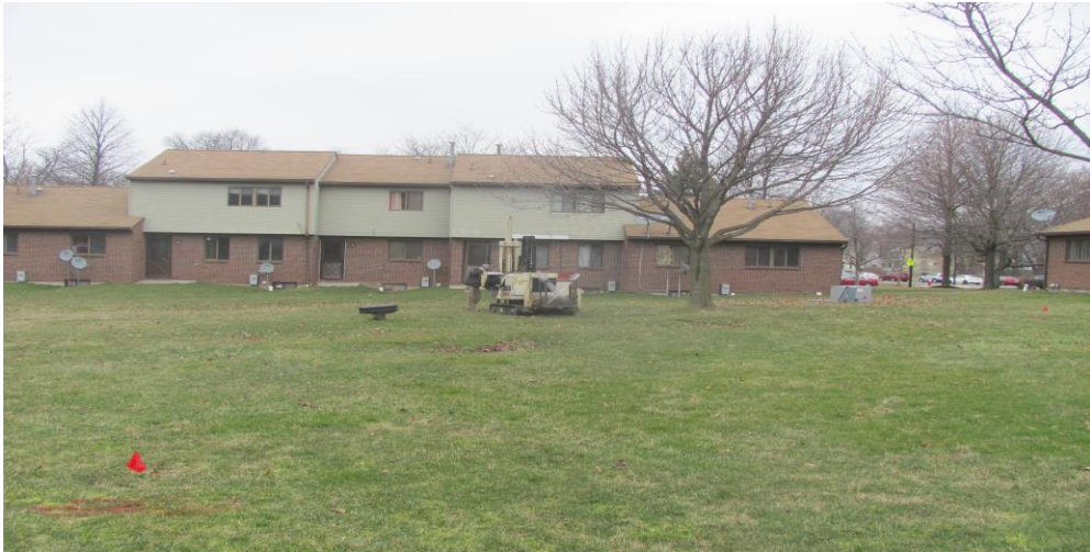
31. Location of Borehole BH-11 from south facing north
