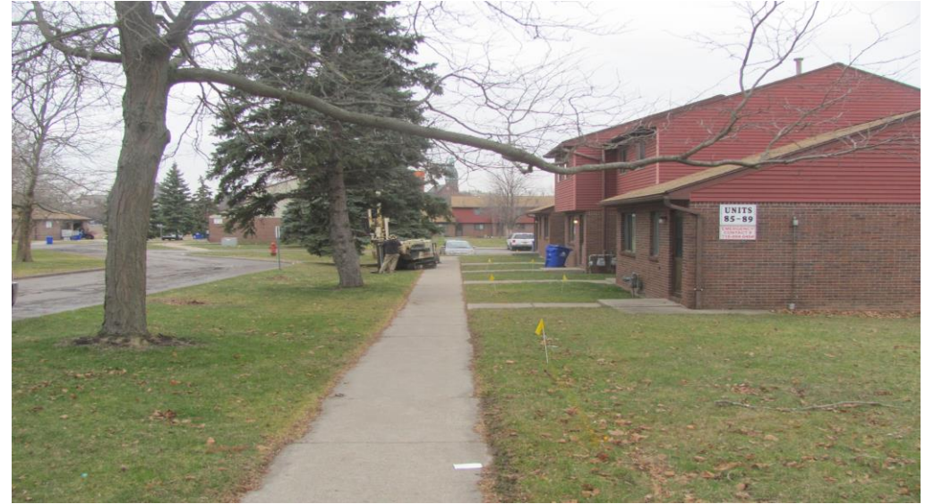
38. Location of Borehole BH-13 from east facing west along Holloway Blvd.
