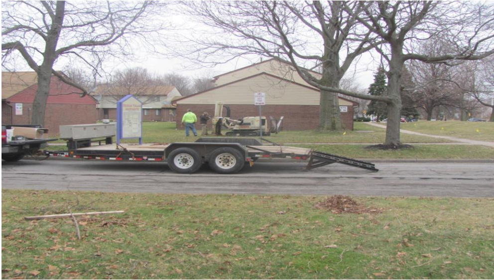
29. Location of Borehole BH-10 from south facing north
