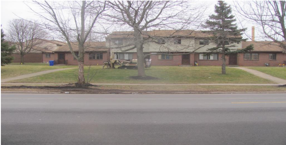
11. Location of Borehole BH-4 from north along Best Street facing south at north end of complex
