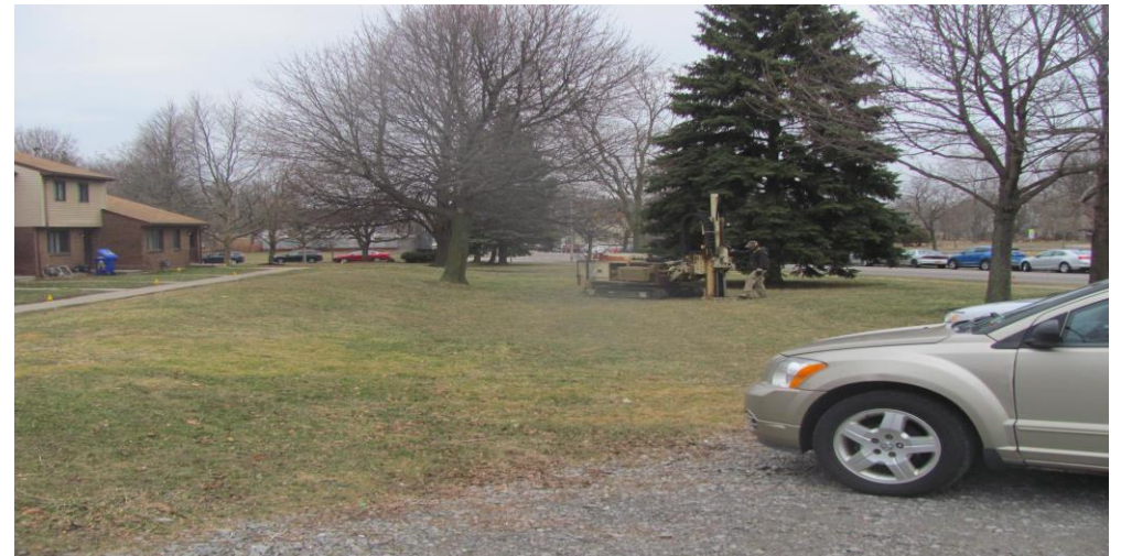
20. Location of borehole BH-7 from south facing north
