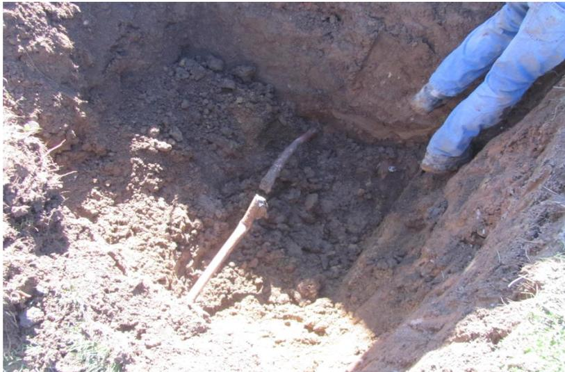
43. BH-22 location, broken copper pipe exposed
