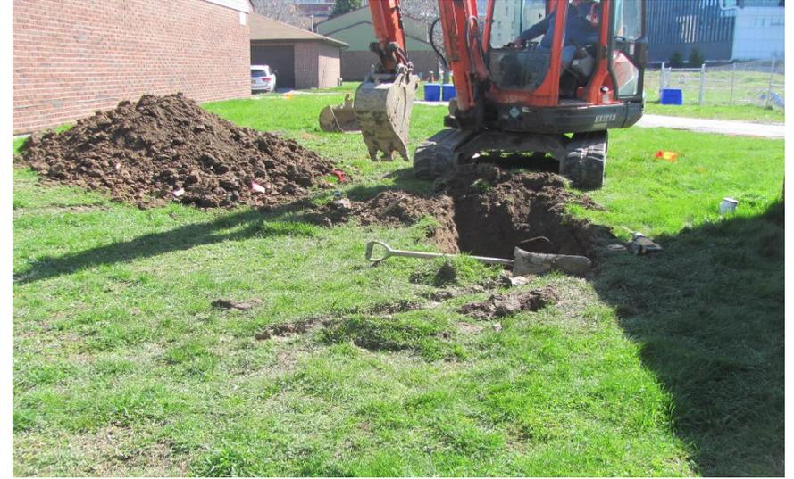
42. BH-22 location, excavator digging to broken pipe
