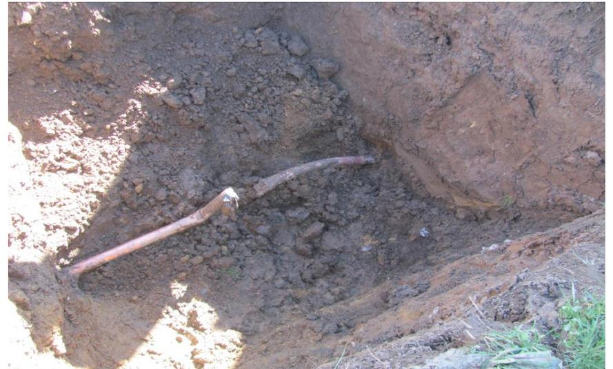
44. BH-22 location, broken copper pipe exposed
