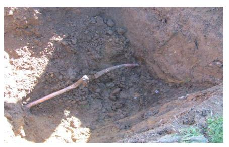
44. BH-22 location, broken copper pipe exposed
