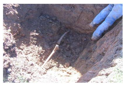
43. BH-22 location, broken copper pipe exposed
