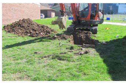
42. BH-22 location, excavator digging to broken pipe
