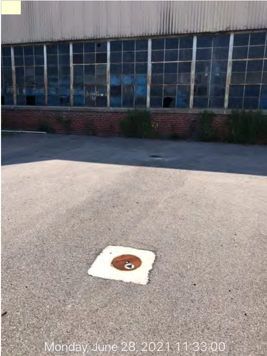
Photo 4: MW in asphalt cover at Former Varnish UST Area
