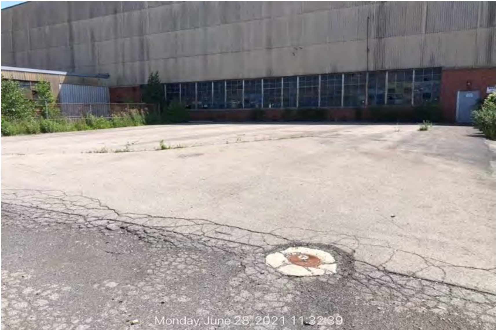
Photo 3: Cover at Former Varnish UST Area
