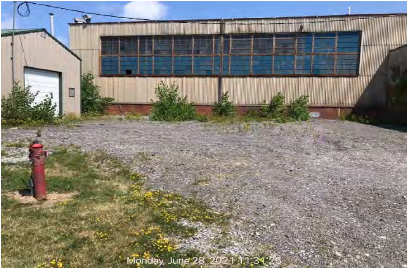
Photo 1: Cover at Former Drum Storage UST Area
