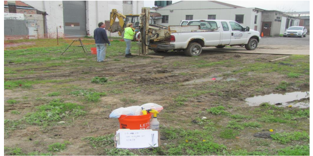
18. Location of Borehole SB-7 from southeast facing northwest
