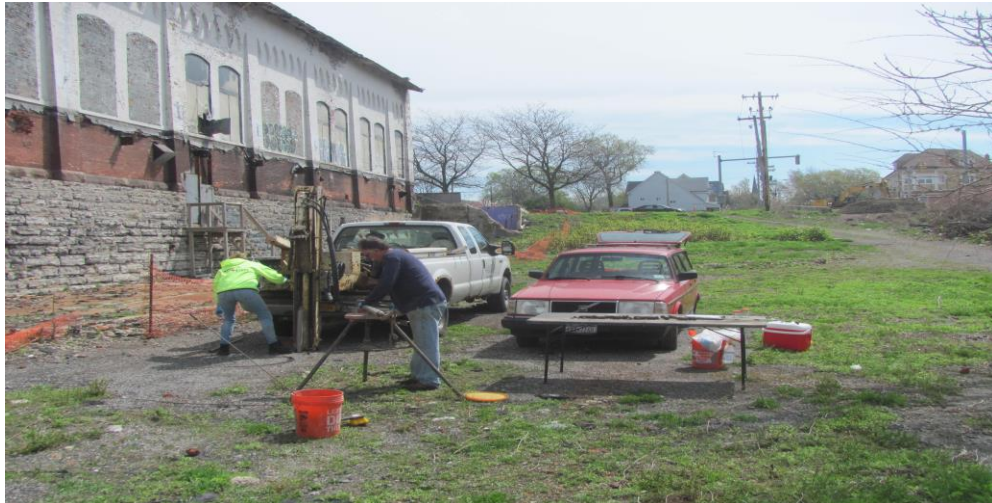
11. Location of Borehole SB-4 from west facing east
