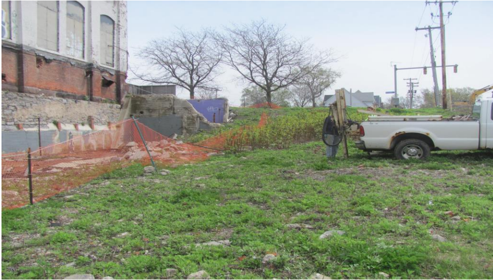
13. Location of Borehole SB-5 from west facing east
