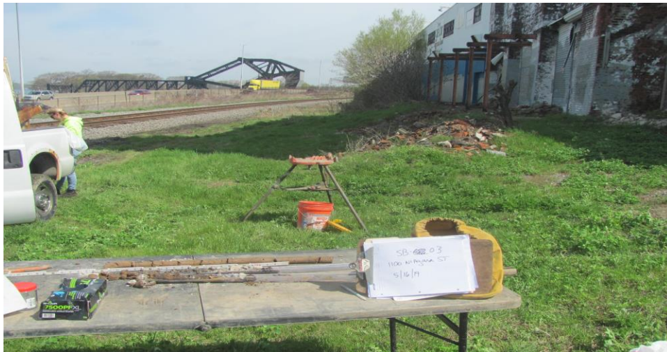
7. Location of Borehole SB-3 from south facing north; located in southwest corner of property
