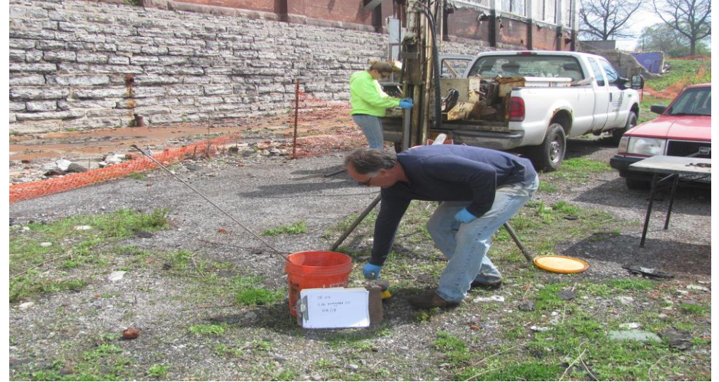
10. Location of Borehole SB-4 from southwest corner facing northeast
