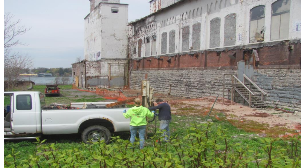
14. Location of Borehole SB-5 from east facing west
