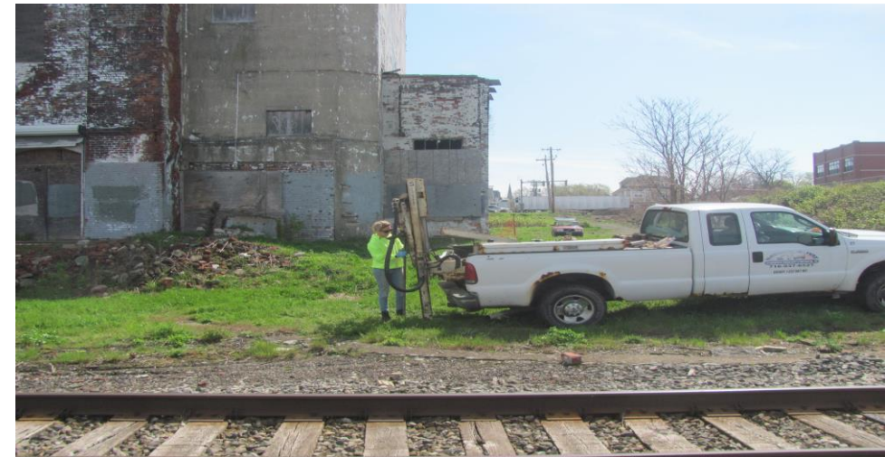
8. Location of Borehole SB-3 from west facing east
