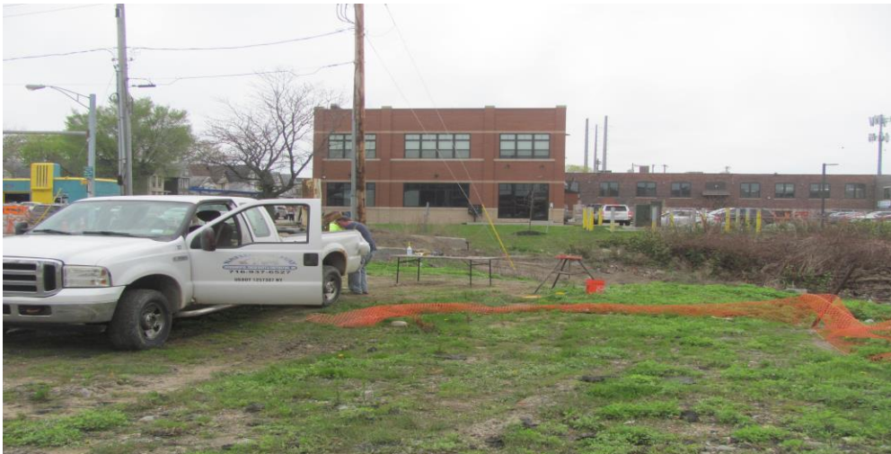
15. Location of Borehole SB-6 from west facing east
