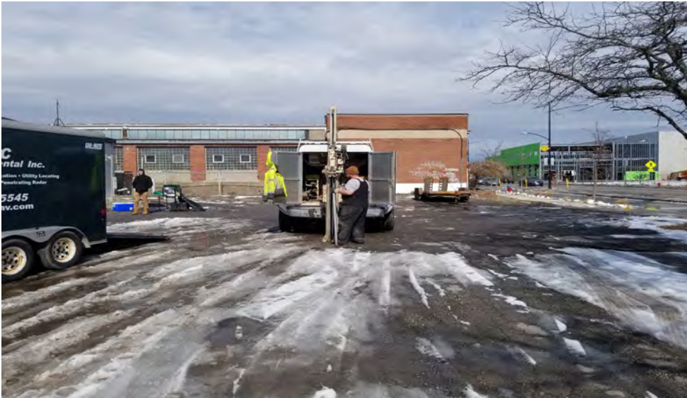
13 BH-5 Location. (Facing North)
