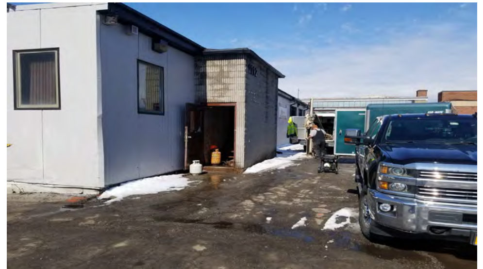
16. BH-6 Location. (Facing North)
