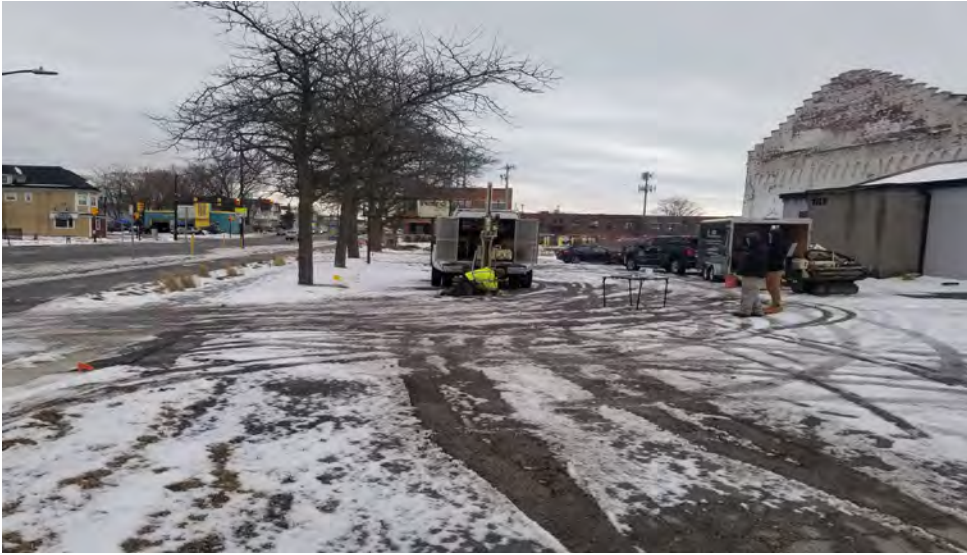
5. BH-2 Location (Facing South)
