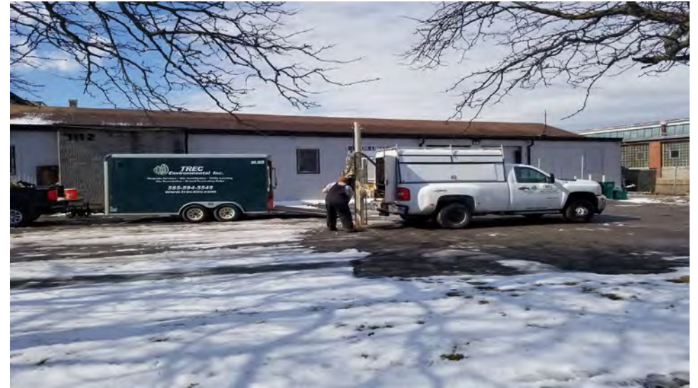
14. BH-5 Location. (Facing Northwest)
