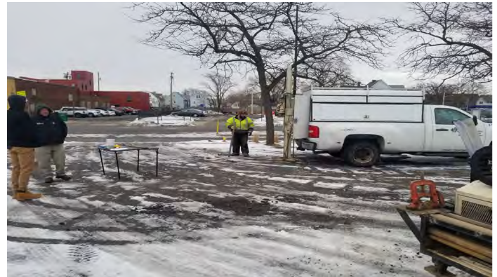
4. BH-2 Location. (Facing East)
