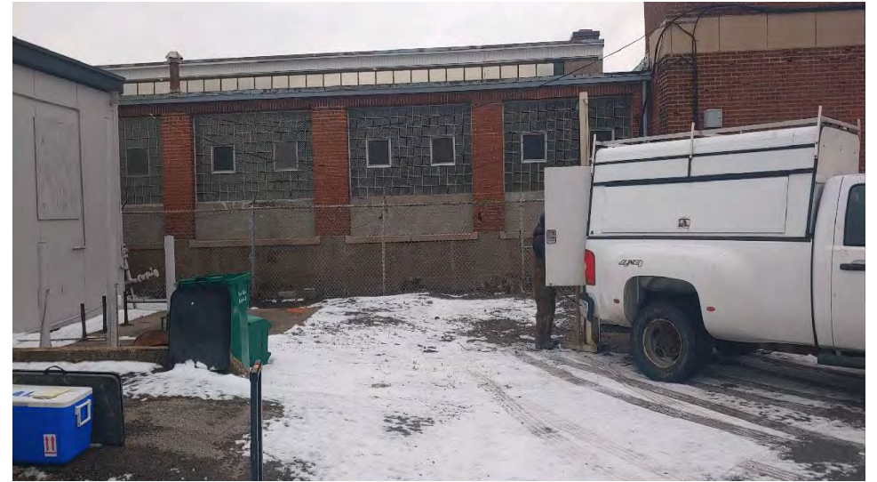
2. BH-1 Location. (Facing North)
