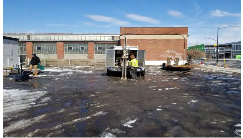
10. BH-4 Location. (Facing north)
