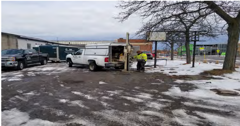
7. BH-3 Location. (Facing North)
