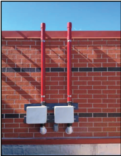
Figure 3.01C: Example of sidewall mounted fans with exhaust stack.
