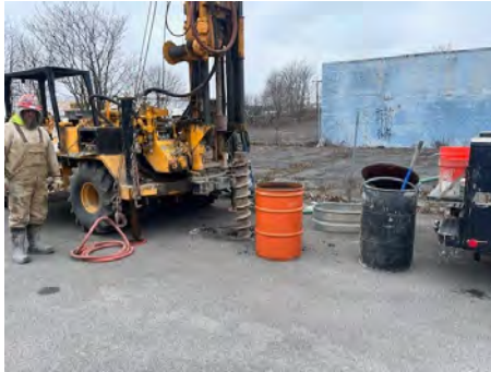
1. Drilling 3' rock socket at RI-MW-3.
