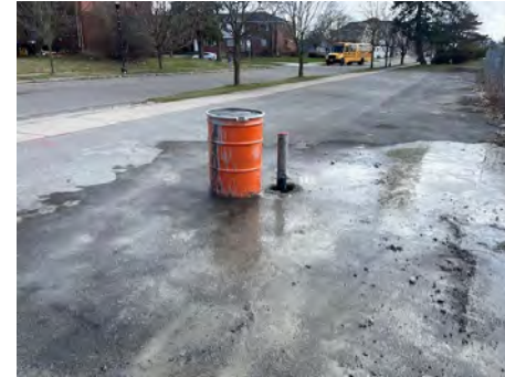
2. Set casing at RI-MW-3.
