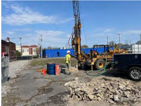
1. Coring additional bedrock at RI-MW-1.
