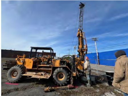
1. Drilling to bedrock at RI-MW-2.
