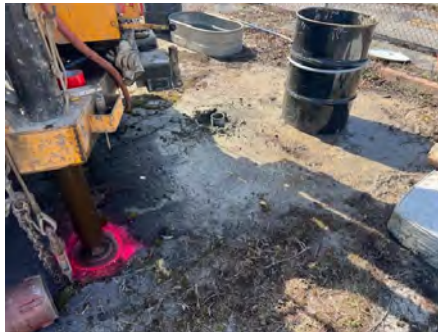
3. Casing set in RI-MW-2.
