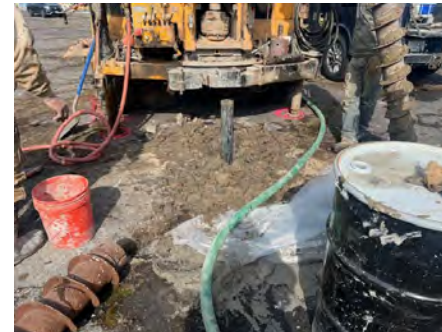
4. Set casing at RI-MW-1.
