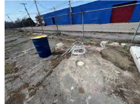
2. Curb box installed at RI-MW-2.
