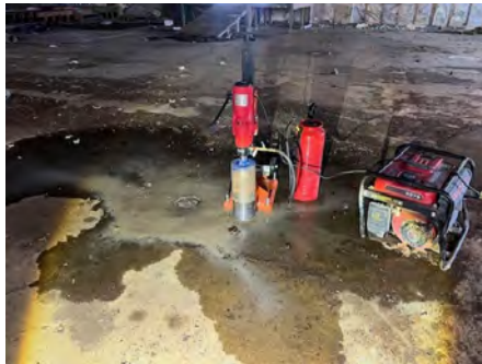
3. Coring concrete at RI-BH-14.
