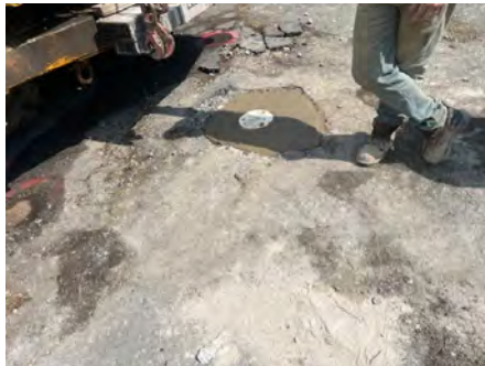
3. Curb box installed at RI-MW-1.
