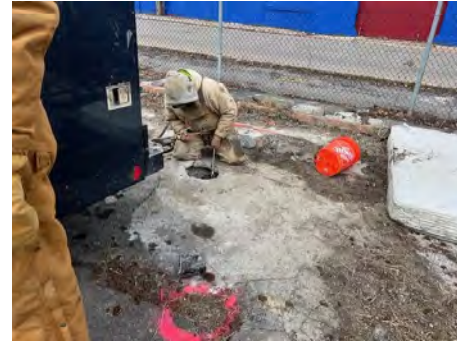
2. Cutting steel casing at RI-MW-2.
