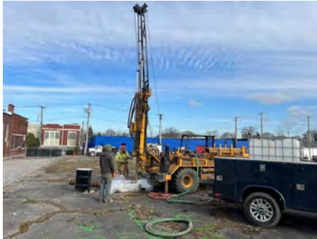
1. Drilling 3' rock socket at RI-MW-1.
