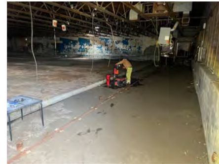
4. Coring concrete at RI-BH-13.
