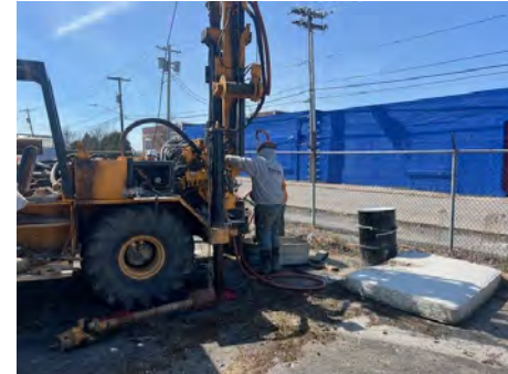
2. Installing casing in RI-MW-2.
