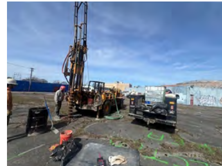
4. Drilling to bedrock at RI-MW-1.
