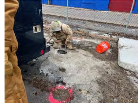
2. Cutting steel casing at RI-MW-2.
