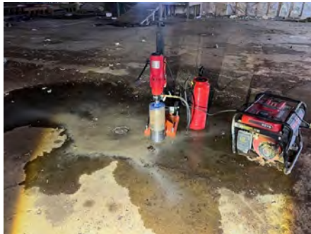
3. Coring concrete at RI-BH-14.
