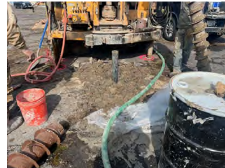
4. Set casing at RI-MW-1.
