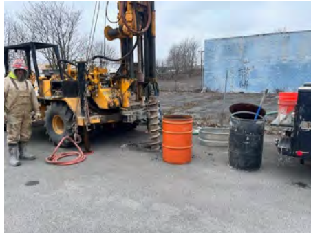
1. Drilling 3' rock socket at RI-MW-3.
