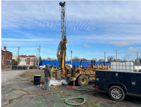
1. Drilling 3' rock socket at RI-MW-1.
