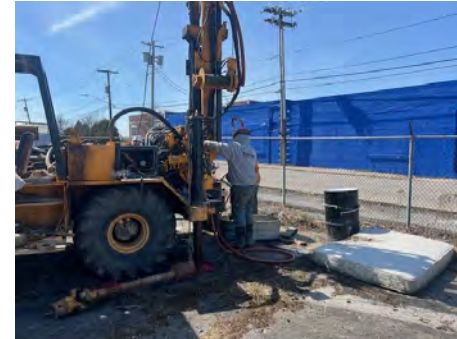
2. Installing casing in RI-MW-2.
