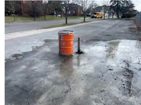
2. Set casing at RI-MW-3.
