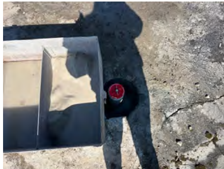
3. RI-MW-2 completed (minus curb box).
