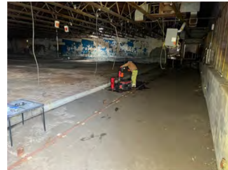
4. Coring concrete at RI-BH-13.
