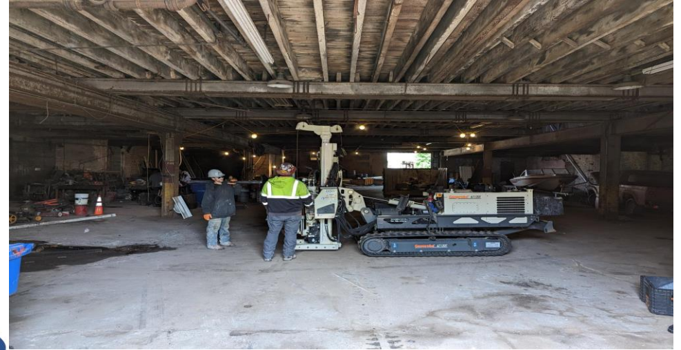
18. Location of BH-7 facing west
