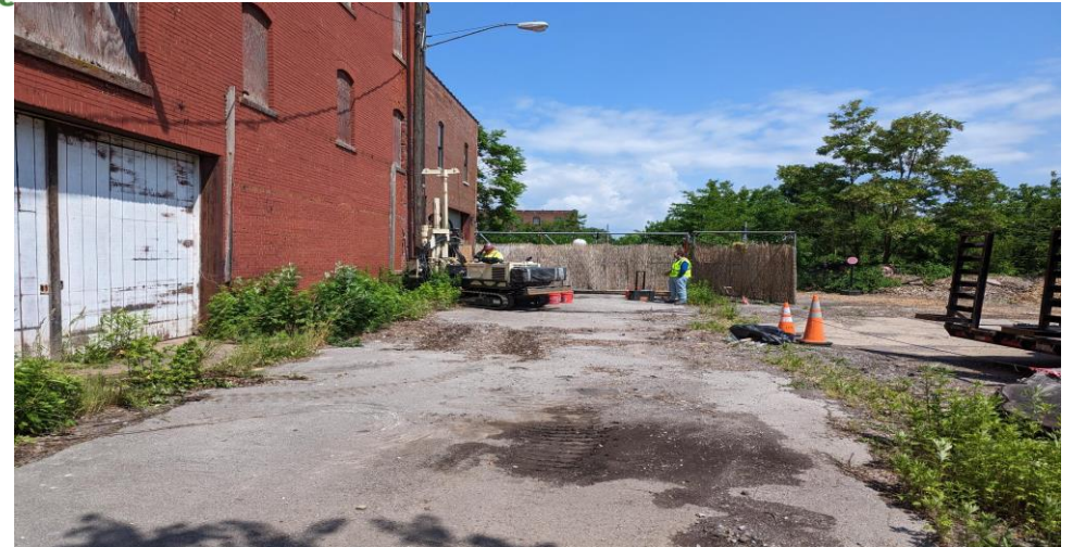
20. Location of Borehole BH-8 facing north
