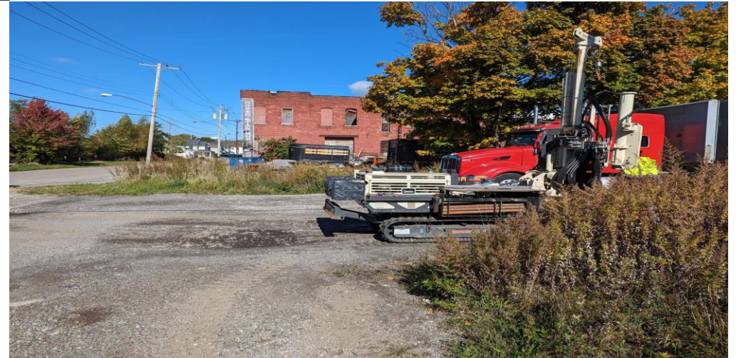
40. Location of BH-14 on 235 Pratt Street facing north.
