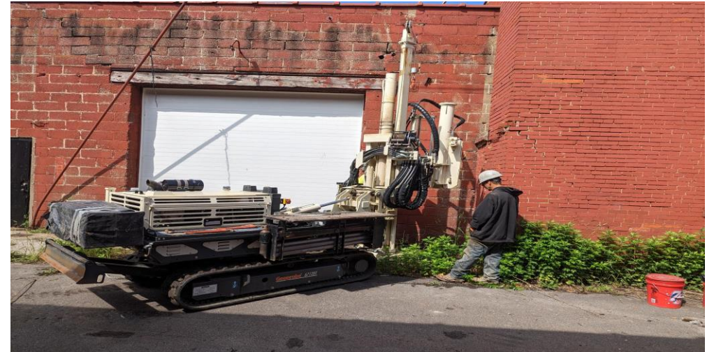
12. Soil Cores from BH-5 facing north
