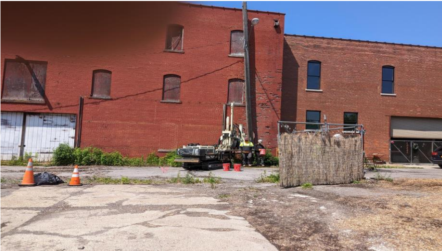
19. Location of Borehole BH-8 location facing west
