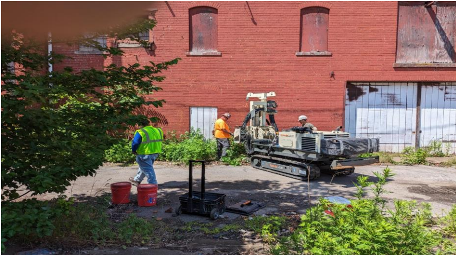
23. Location of Borehole BH-9 facing west
