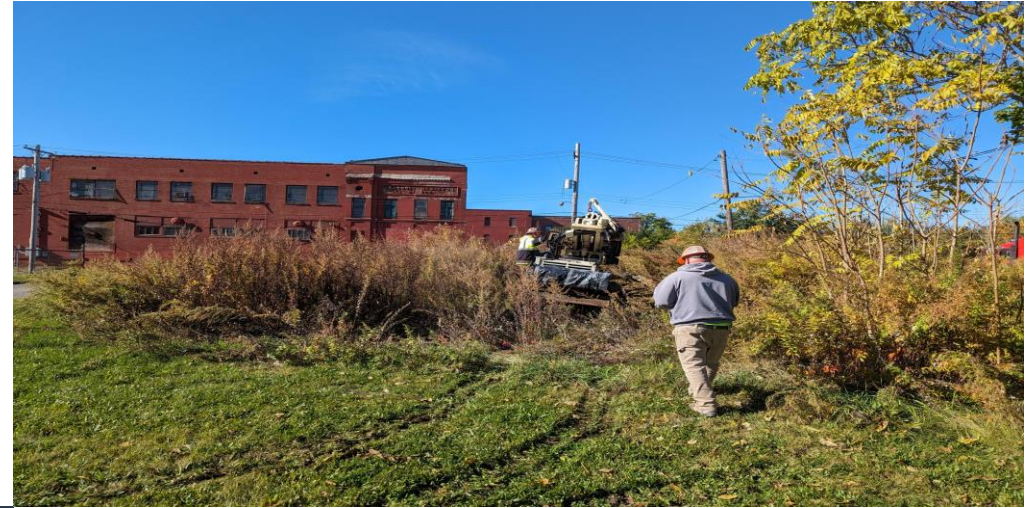
30. Borehole BH-11 on east end of 231 Pratt Street facing west
