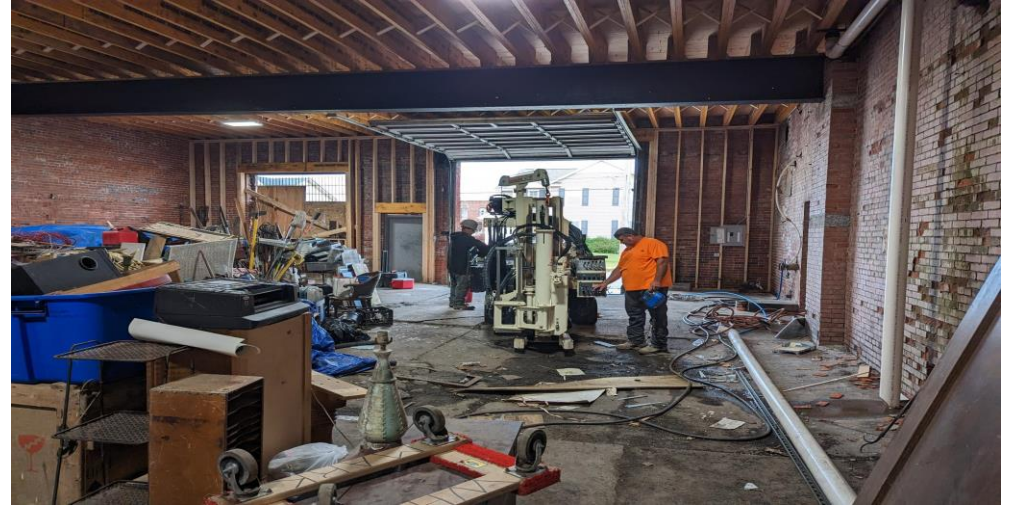
2. Location of Borehole BH-1 facing west
