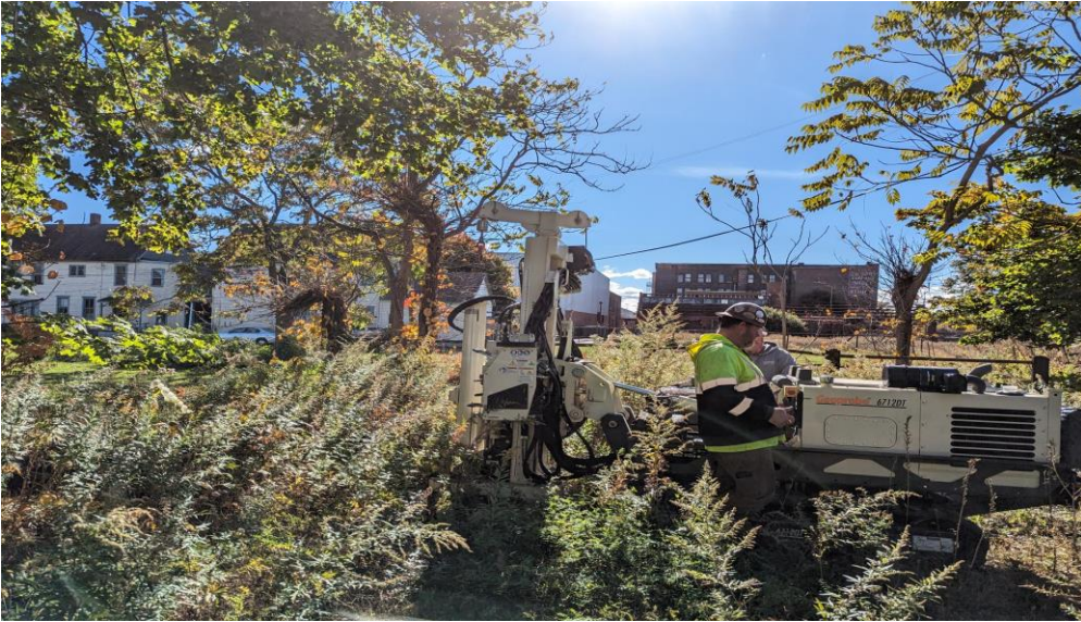
37. Location of BH-13 on 235 Pratt facing south.
