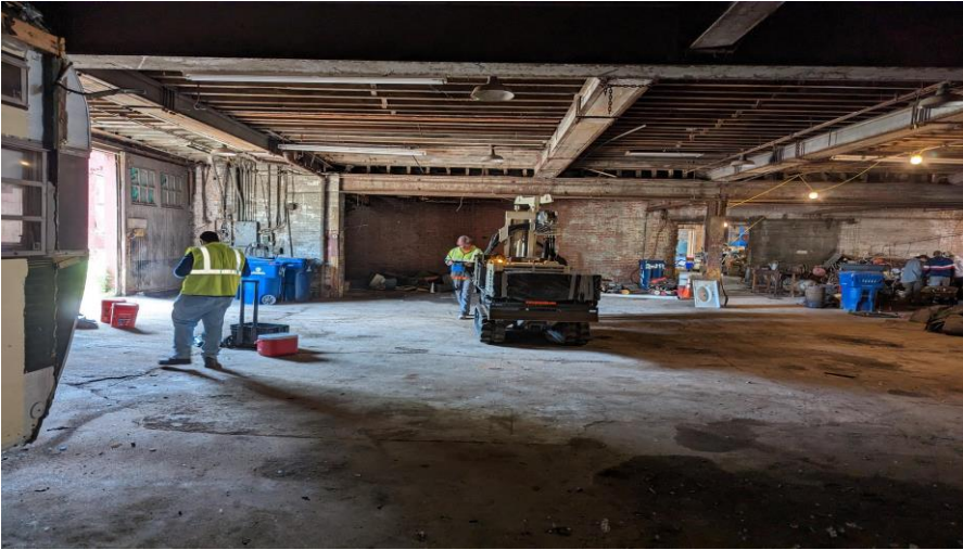
17 Location of Borehole BH-7 facing west
