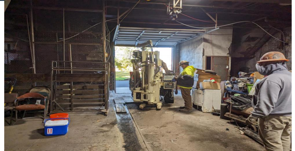
4. . Location of Borehole BH-02 middle west in 273 Hickory Street
