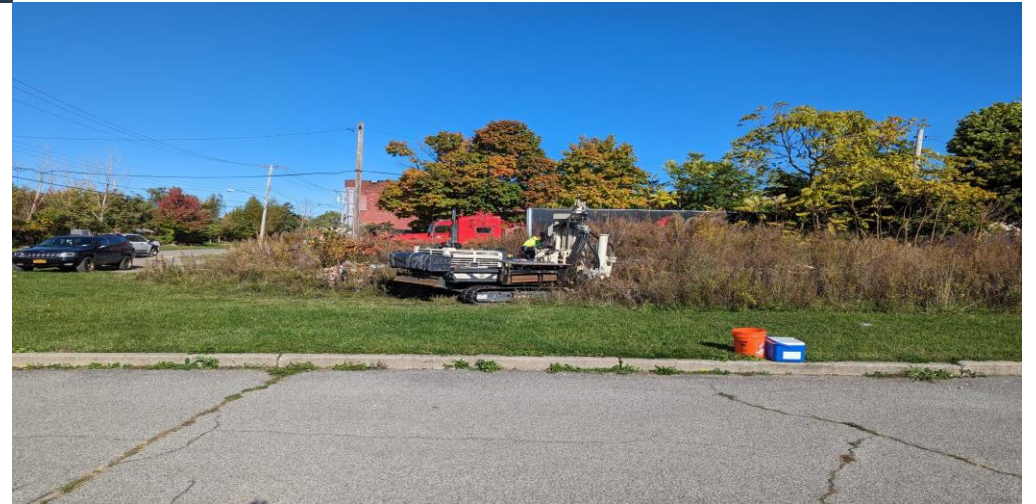
24. Location of borehole BH-09 on 229 Pratt Street facing north
