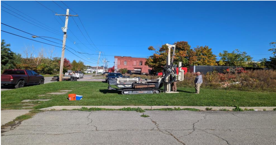
23. Location of BH-08 on 229 Pratt Street facing north
