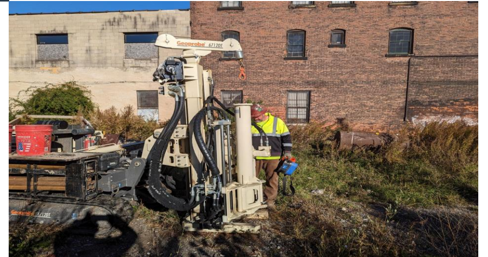
16. Location of Borehole BH-06 eastern end of 337 Hickory Street parcel
