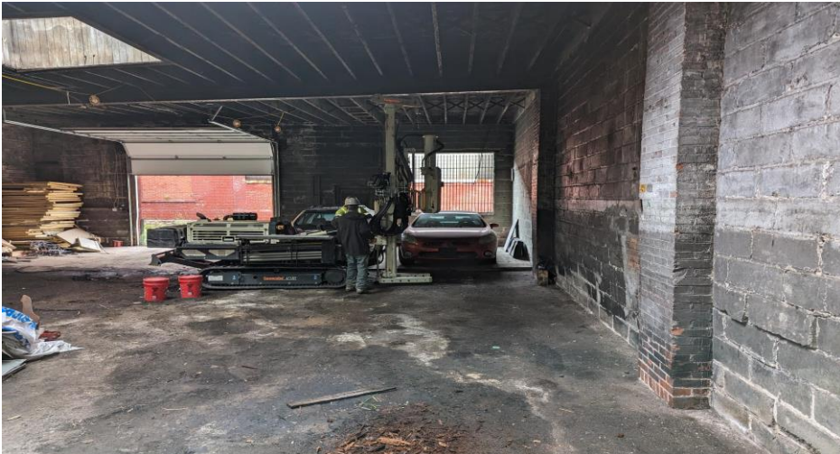
7. Location of BH-3 facing east
