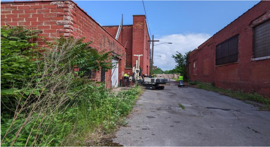
13. Location of Borehole BH-5 facing north
