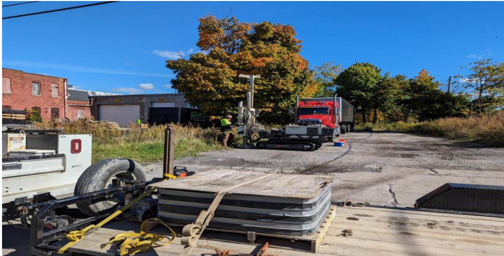
43. Location of Borehole BH-15 on northwest side of 235 Pratt Street facing east from Pratt Street
