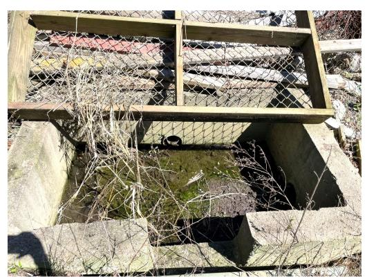
Photograph 5: Suspected concrete rinsing pit, grated top was originally over the concrete pit. Removed the grated top to collect a sample of the sediment material within the pit (SED-1). This structure is located in an apparent former storage area (top of photo is north).
