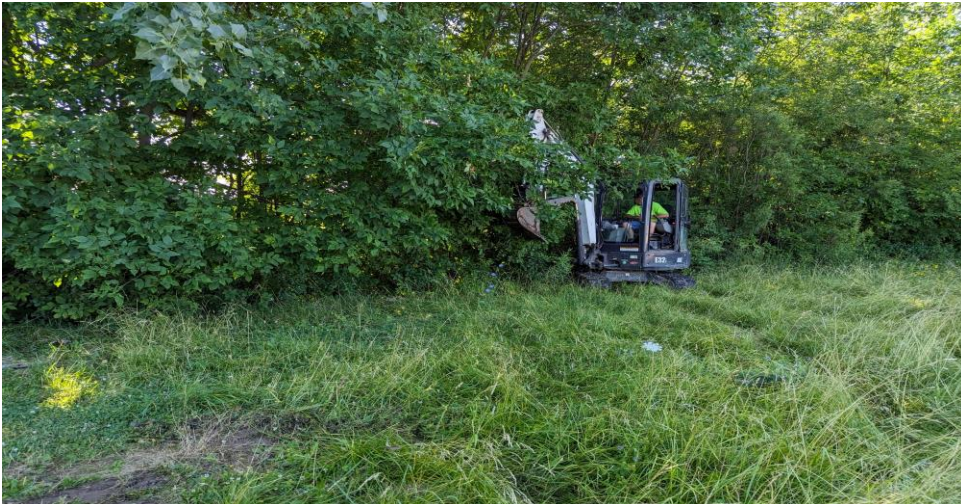
15. Location of Test Trench 8 (TP-8) facing southeast
