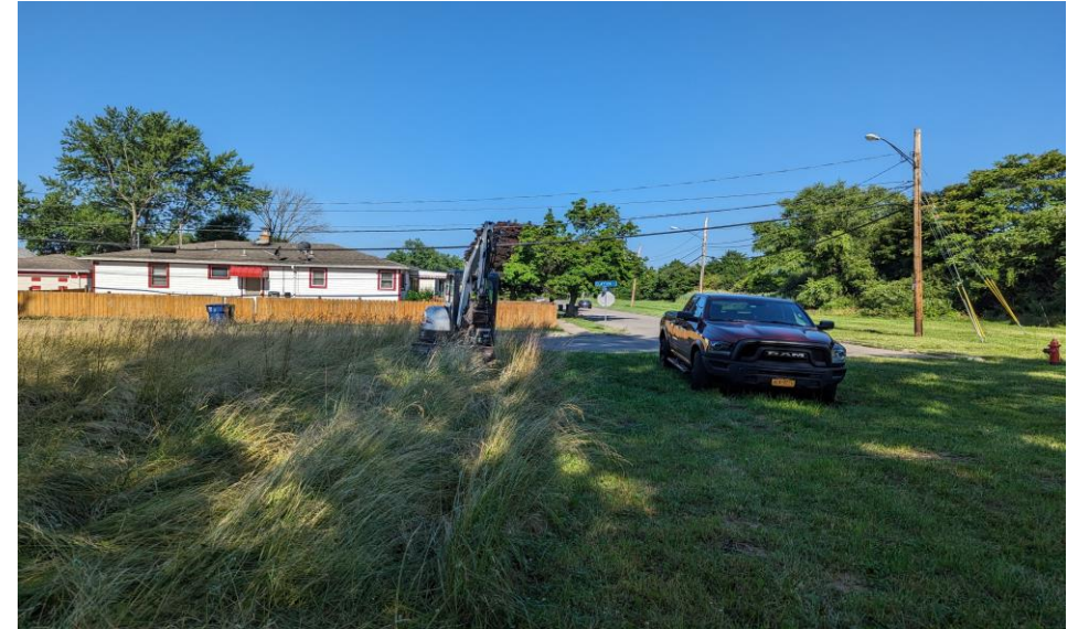
14. Location of Test Trench 7 (TP-7) facing west
