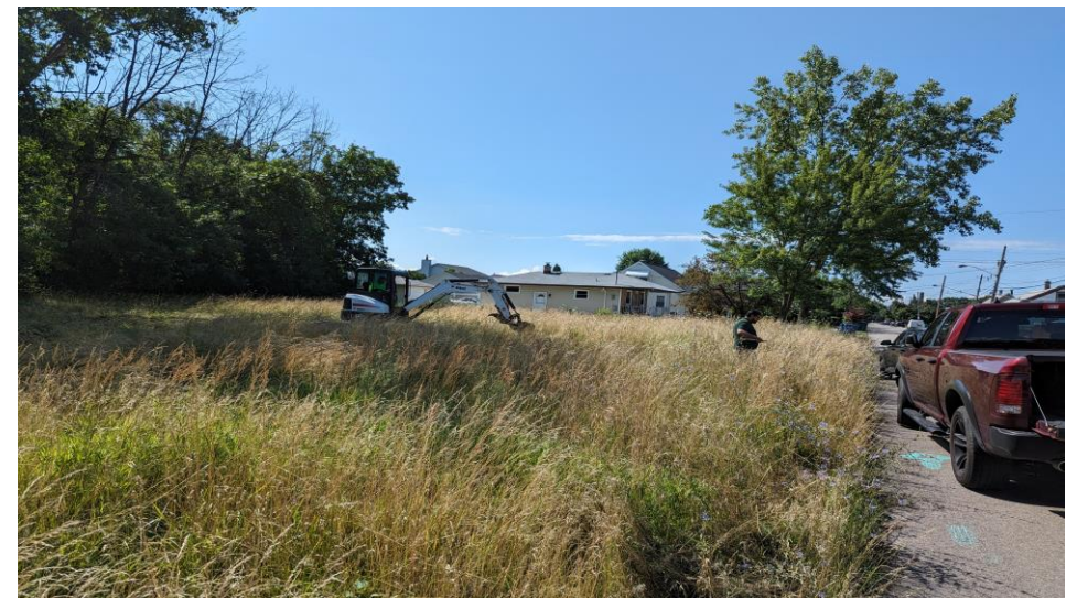
20. Location of Test Trench TP-11 facing south
