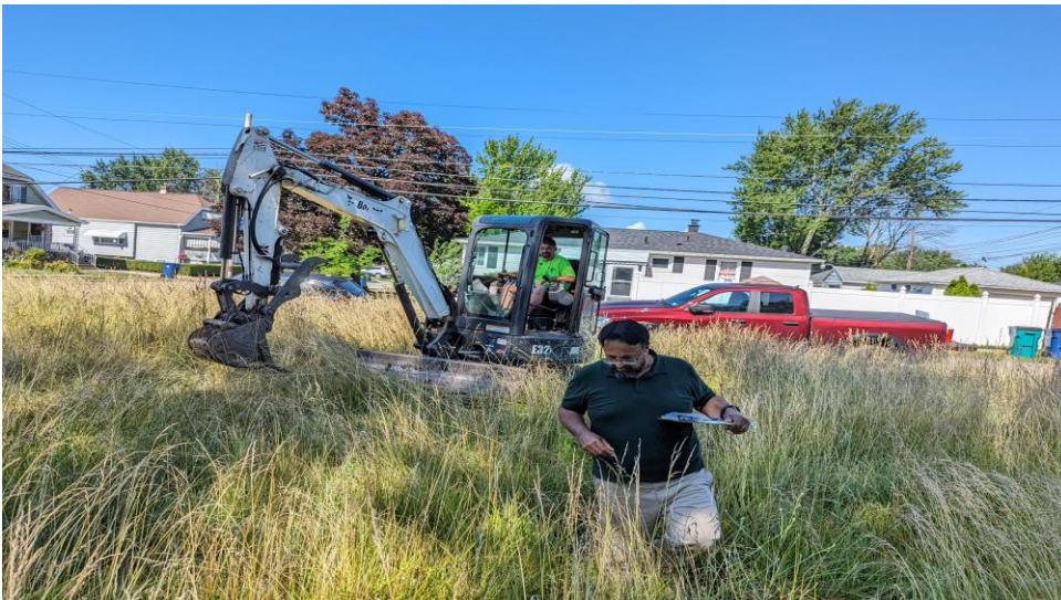
19. Location of Test Trench 11 (TP-11) facing west
