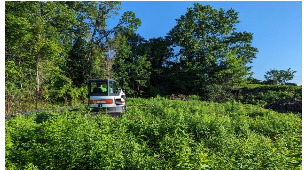
4. Location of Test Trench TP-2 facing north
