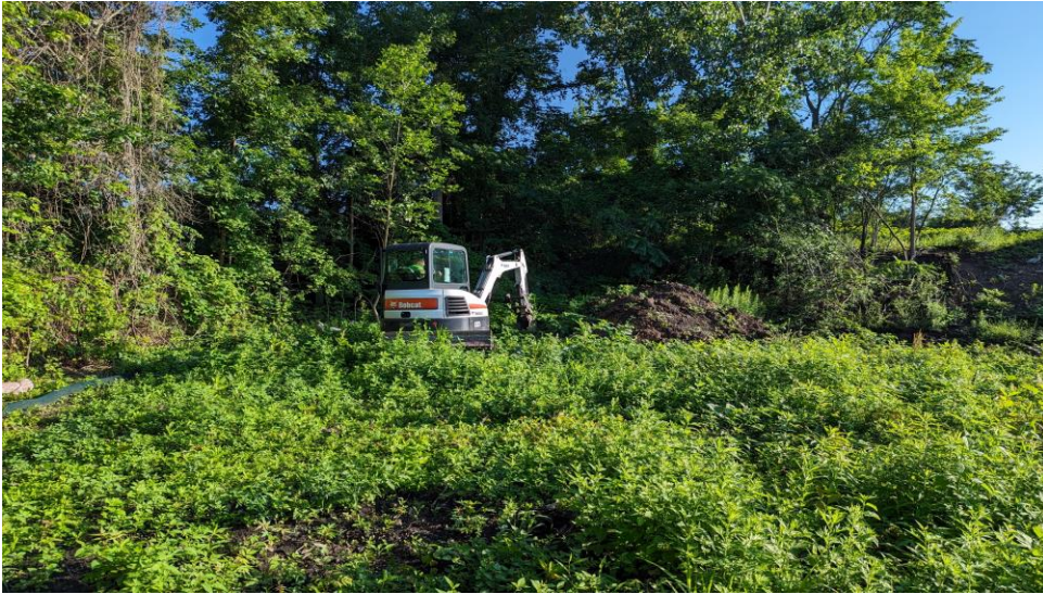
1. View of Test Trench 1 (TP-1) facing north (in northeast corner)
