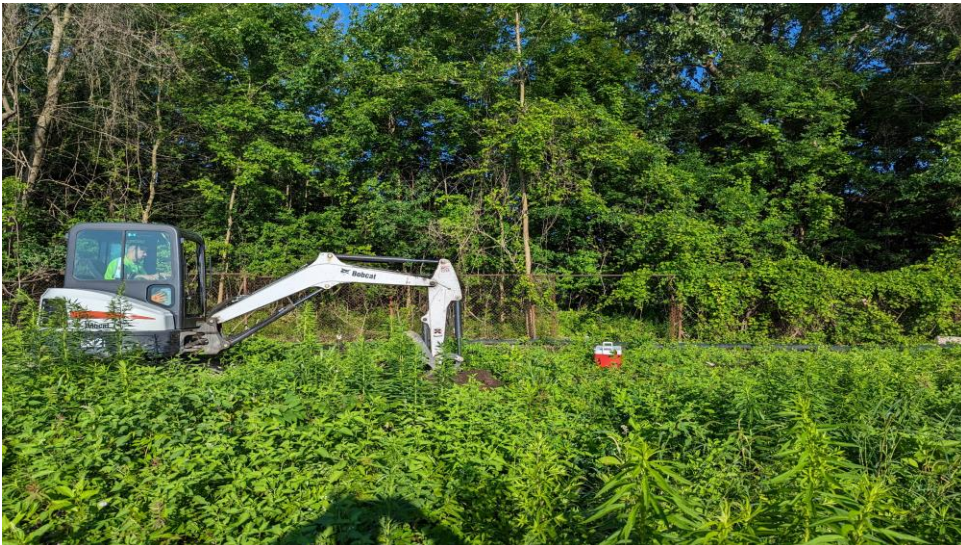
3. Location of Test Trench 2 (TP-2) facing west
