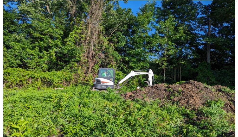
2. Location of TP-1 facing west
