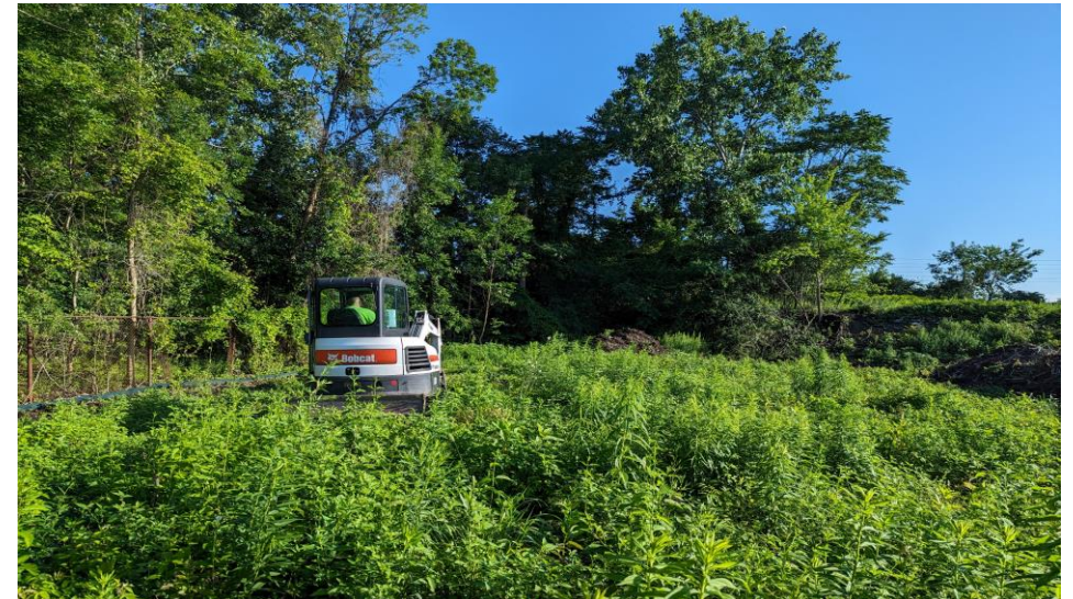
8. Location of Test Trench TP-3 facing north
