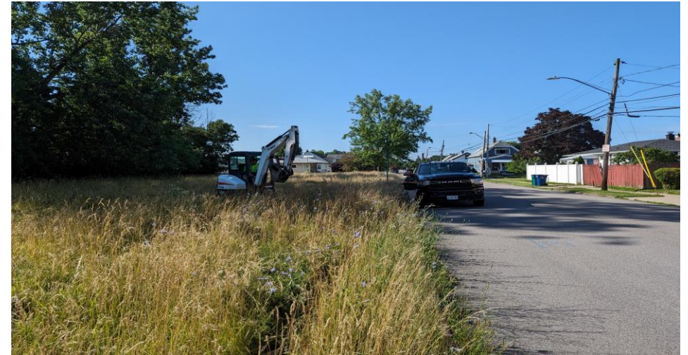
16. Location of Test Trench TP-9 facing south
