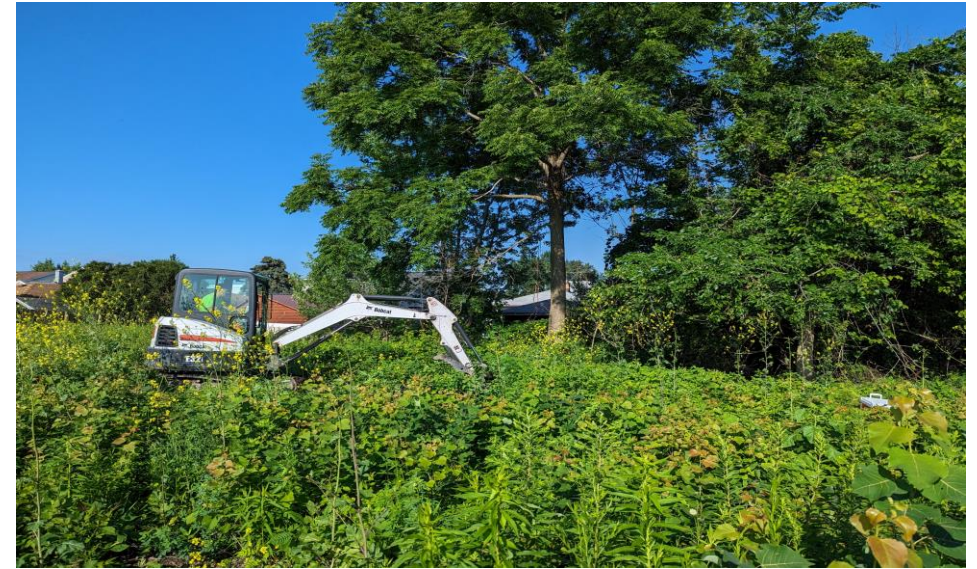
10. Location of Test Trench 4 (TP-4) facing southwest
