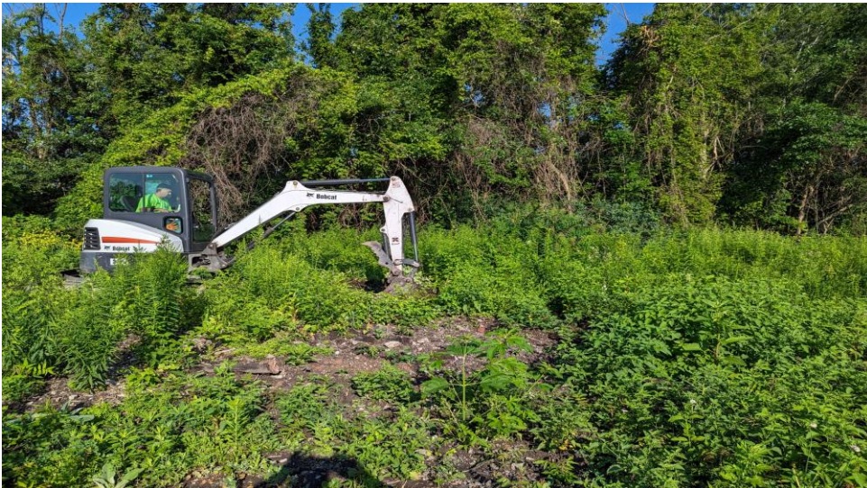
7. Location of Test Trench 3 (TP-3) facing west
