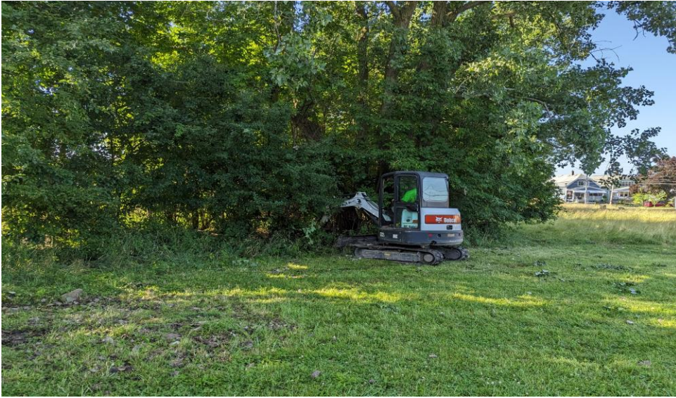
13. View of location of Test Trench 6 (TP-6) facing southeast
