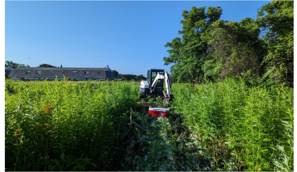
6. Location of Test Trench 3 (TP-3) facing south
