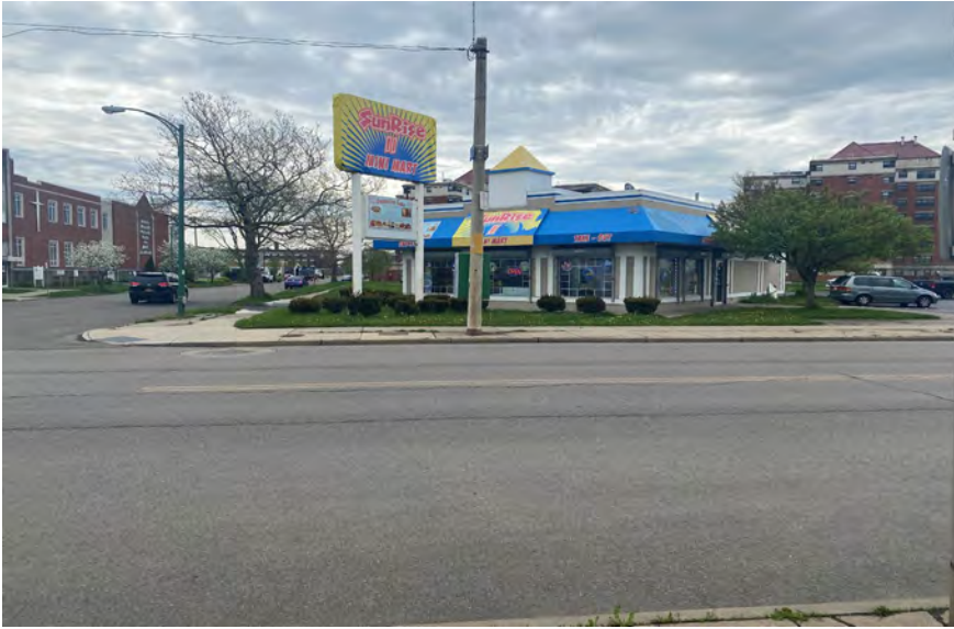
5. Northwest corner – west facing east
