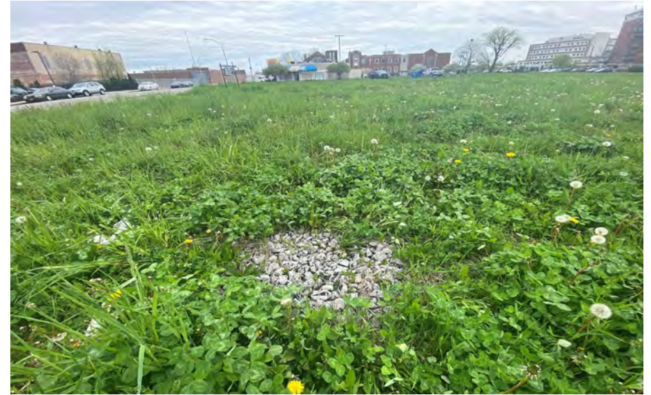
14. Typical gravel seen in various locations across property
