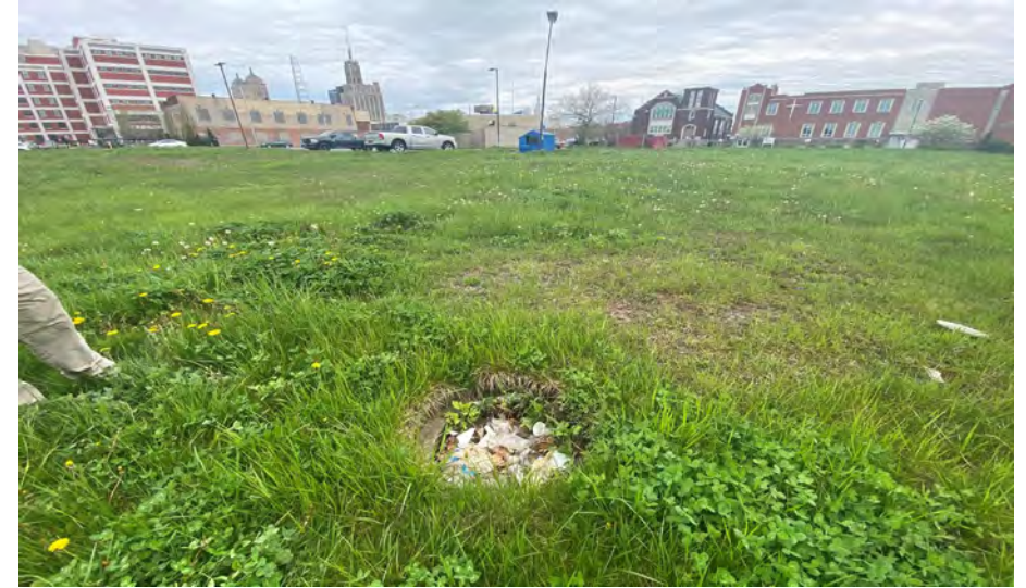
10. Old sewer drain on northeast corner of lot
