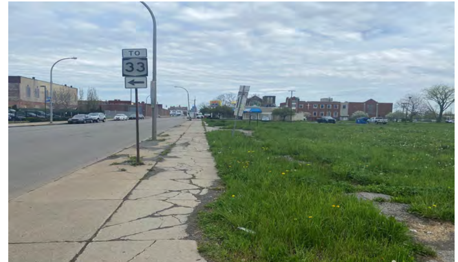
16. South facing north, along western border of property
