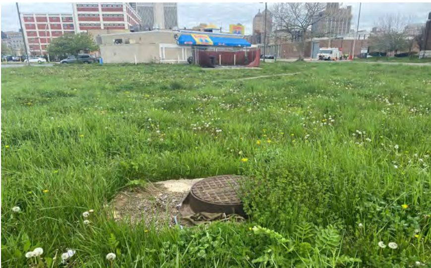
11. Sewer line/man hole – northeast corner
