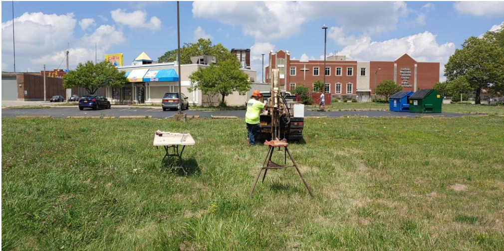
23. Location of Borehole BH-8 from south facing north
