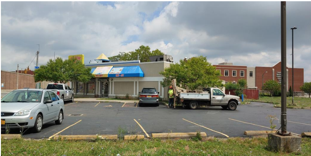
15. Location of Borehole BH-5 from south facing north
