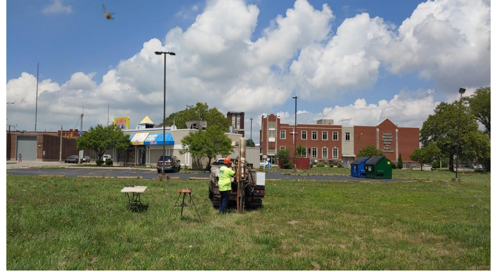
22. Location of BH-7 from south facing north
