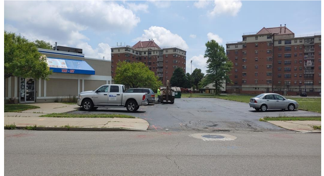
14. Location of Borehole BH-5 from west facing east
